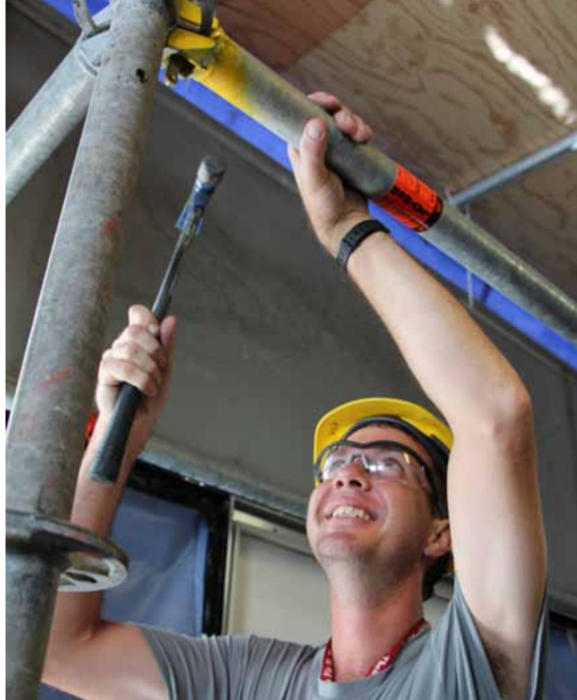
Code 970 Shipwright Apprentice Charles Chang - Humphreys tightens brackets on staging for USS Halsey (DDG-97.)
