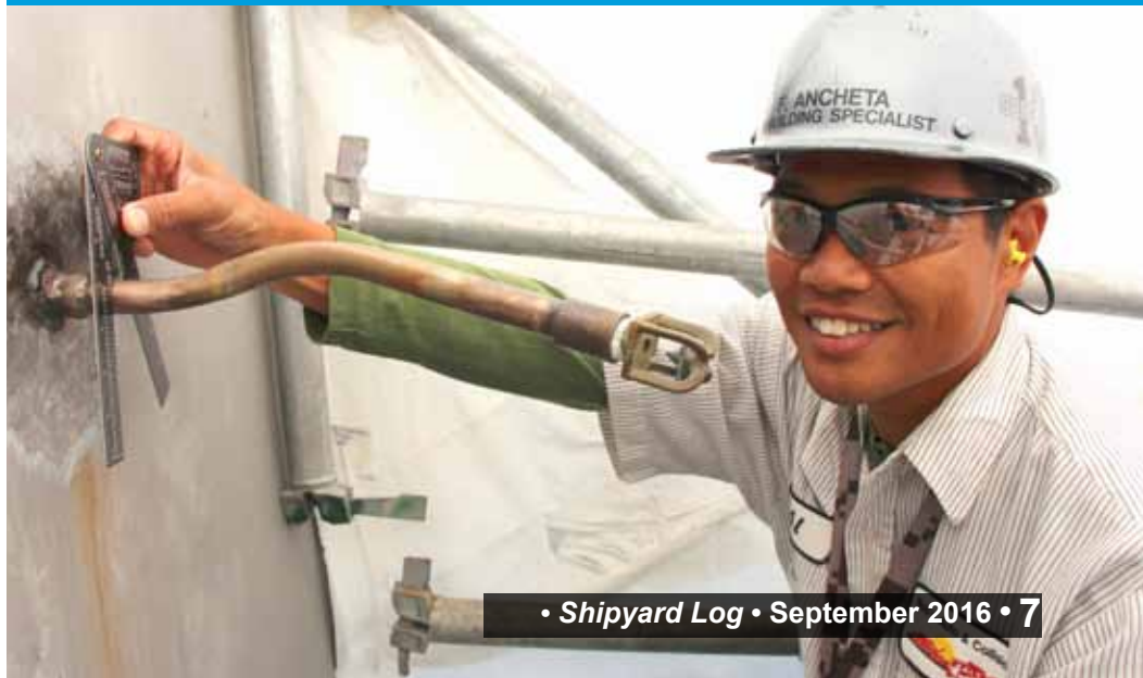
Code 103 Shipbuilding Specialist Freddie Ancheta measures a Counter Measure Waste Down piping, to verify completed contractor work on USS Halsey (DDG-97.)
