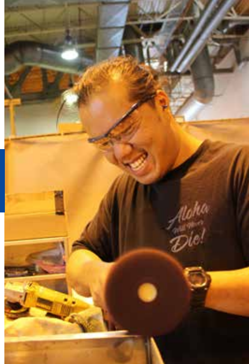
Code 920 Sheet Metal Mechanic Robert Seronio works on a sheet metal locker cover for a trash disposal unit in support of USS Texas (SSN – 775.)
