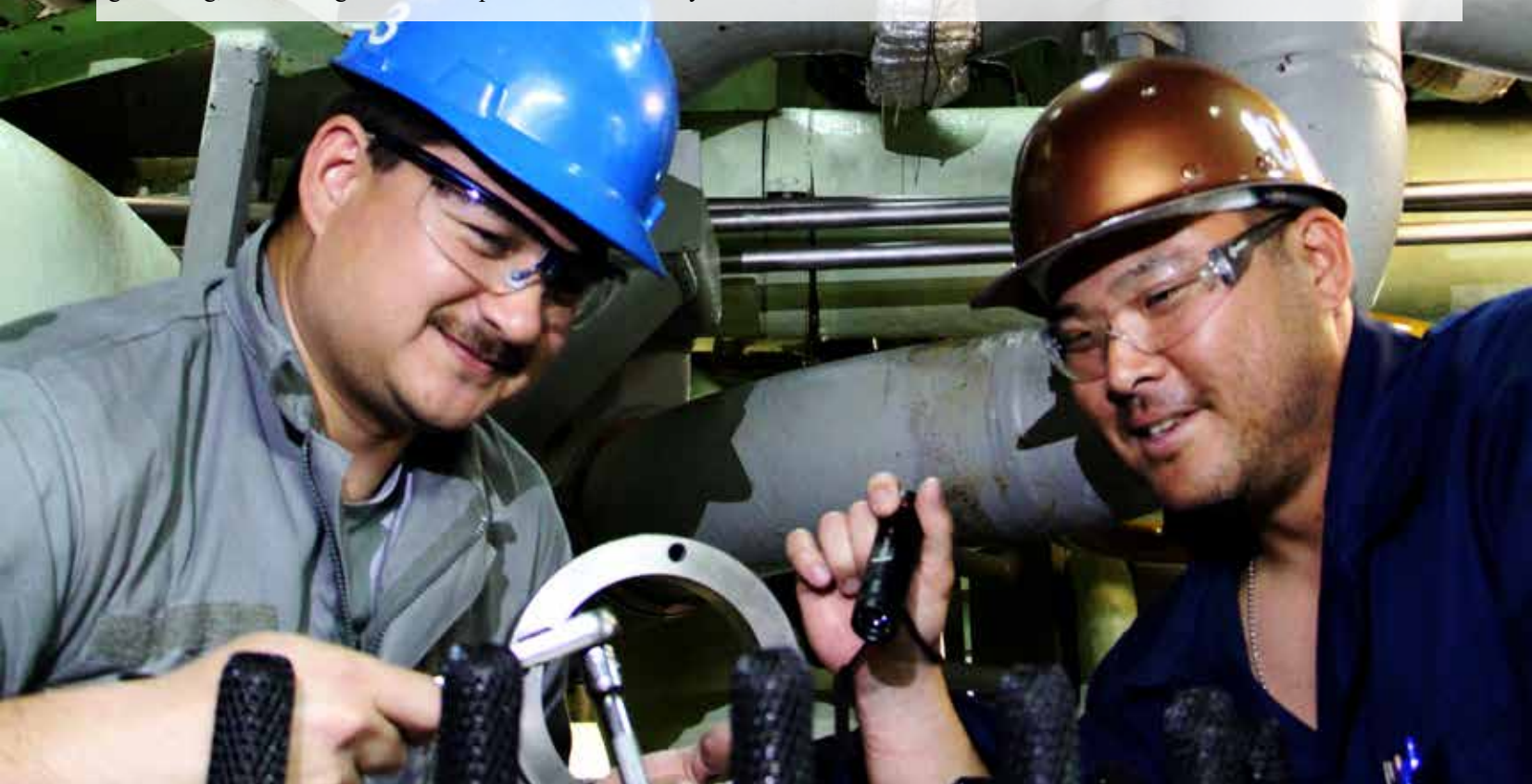
Shop 38 Machinist Apprentice Geoffrey Kop and Code 133 Marine Machinery Inspector Leader Wade Taguchi perform a “controlled fit-up” of a mechanical seal on a seawater pump during a recent submarine availability. Controlled fit-ups require Code 133’s presence to ensure the correct material is installed and the fit-up is performed in accordance with all applicable requirements.
