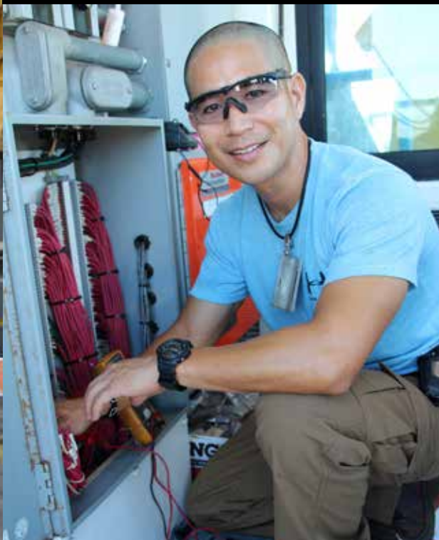
Code 730 Electrician work leader Landon Nakayama routes new wiring through the Travel Systems Alteration in the Operator's cab.
