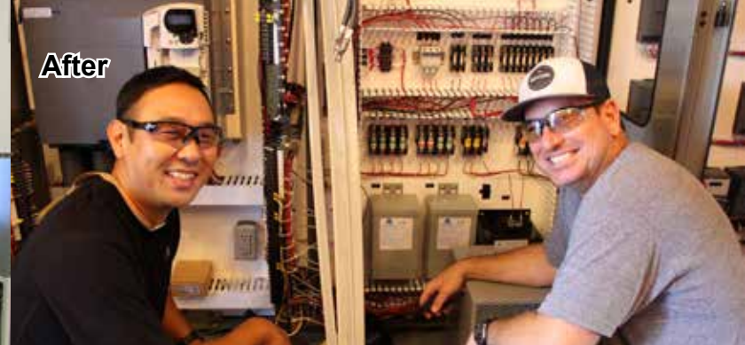
Code 730 Electrician work leader Shaun Murakami and Electrician Mechanic Tom Talkington put the final touches on the total overhaul of the Travel Drive Systems on Portal Crane P-81.
