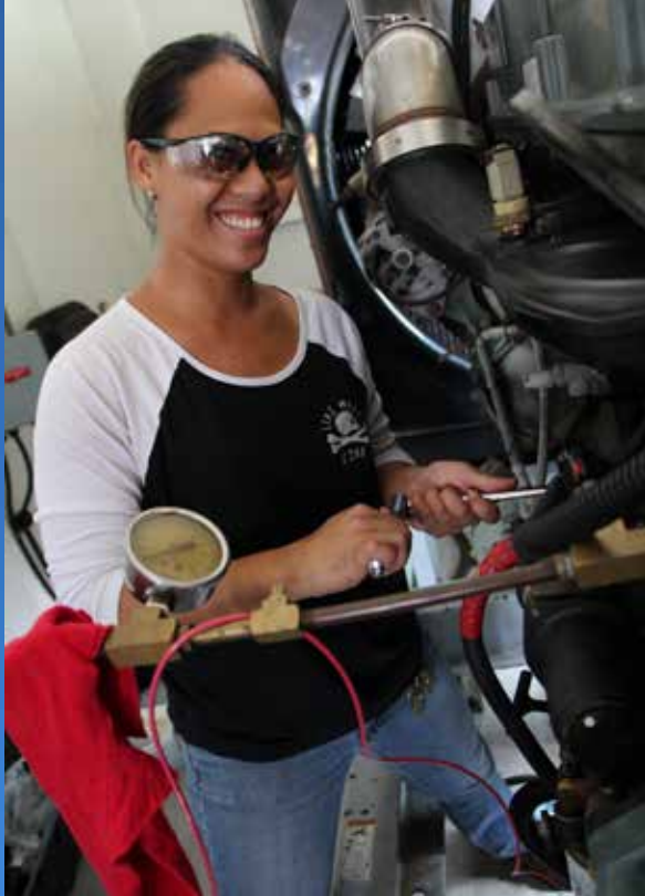
Code 730 Electrician Apprentice Tanya Labajo performs electrical maintenance on portal cranes which provides efficient lifting capabilities for heavier items.
