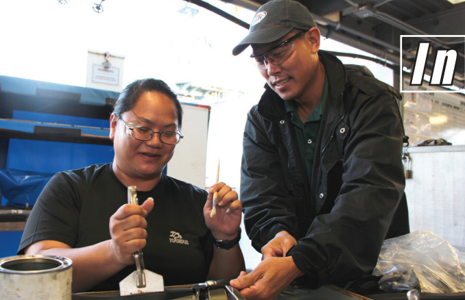
Shop 17 Supervisor Wayne Kamikawa provides oversight to Shop 17 Workleader Katherine Himoto as she installs new gaskets onto a switchboard cover. The purpose of the gaskets is to keep water and debris out of the switchboards.
