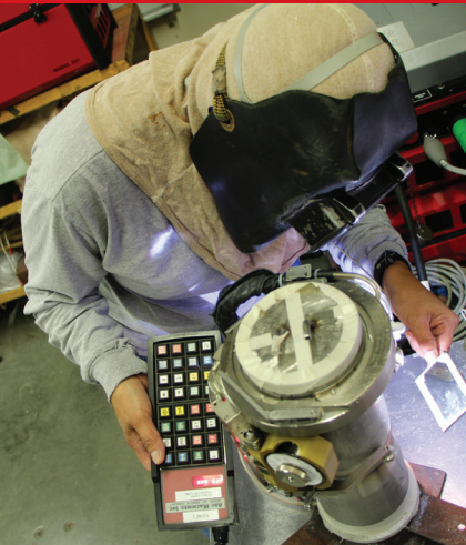
Shop 26 Welder Mechanic Bernie Manibog operates the Arc Machine Incorporated (AMI) mechanized pipe welding machine.
