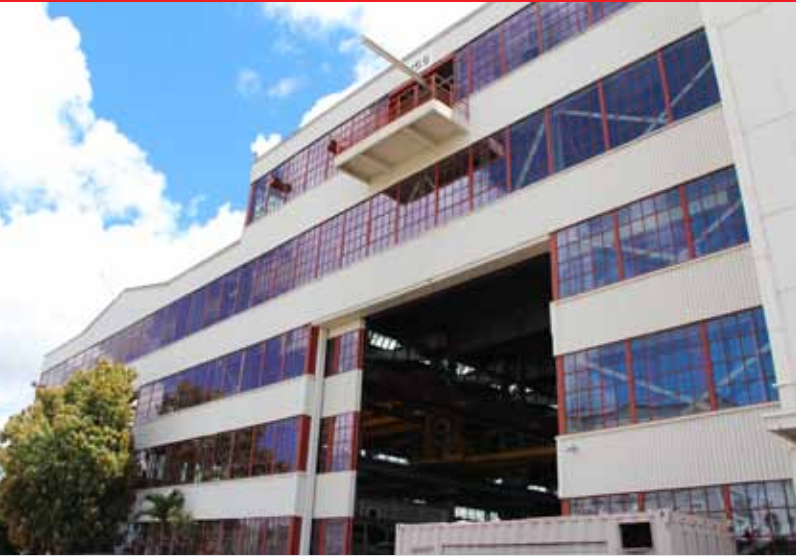
2014 Preservation Honor Award: Building 155 Rehabilitation Awardees: Hope's Windows; JBPHH; Mason Architects, Inc.; CNRH; NAVFAC Hawaii; PHNSY&IMF and Code 1160
