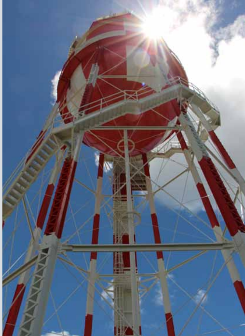
2015 Preservation Honor Award: Waterfront Operations Signal Tower Rehabilitation Awardees: PHNSY & IMF; NAVFAC Hawaii
