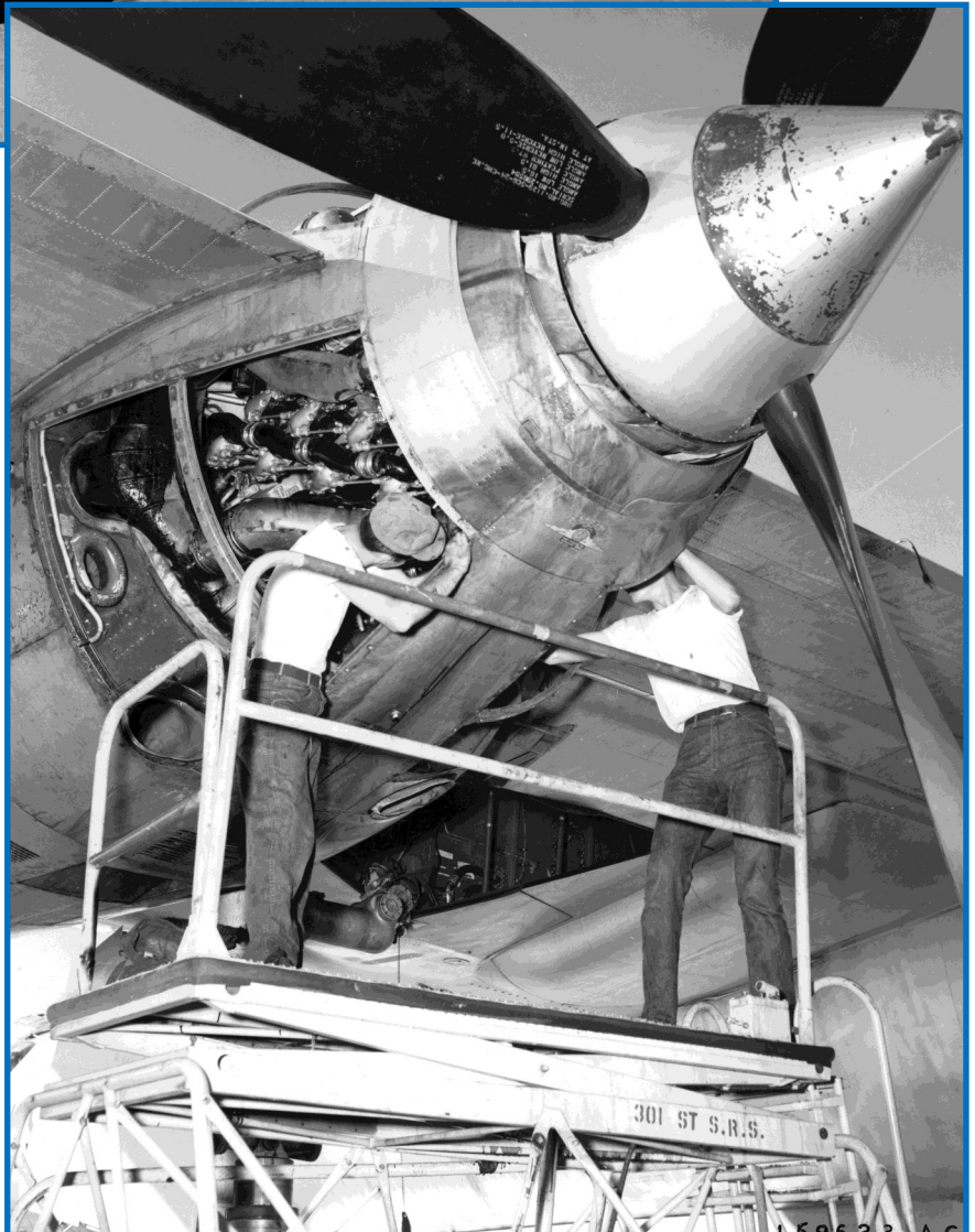
Top: Air Force enlisted maintenance technicians perform hands-on training for the Pratt & Whitney R-4360 engines in the B-36.
