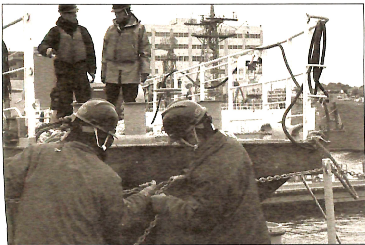
Crew members from the carpenter shop connect chains for the fences on caisson No. 4 to prepare for moving the vessel.
