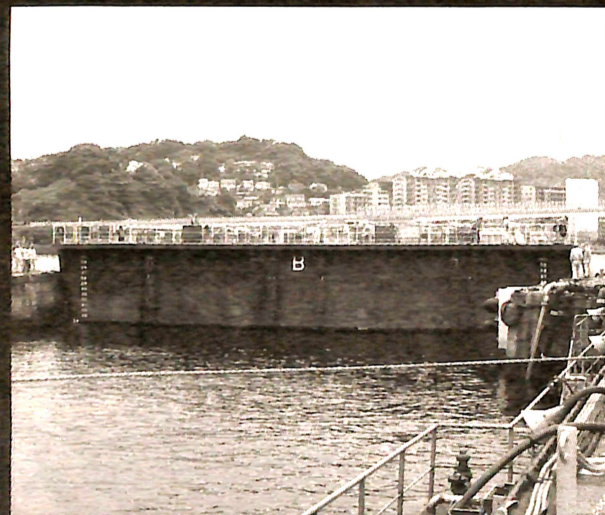
Once the ship is held in position with the lines and the pusher boats have exited the dry dock, the caisson is closed.
