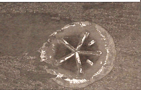
(top) A worker applies the final coat to a tiedown fitting inside a tent built on the flight deck of USS Kitty Hawk (CV 63). (bottom) A tiedown fitting and surrounding non-skid coat that are worn down after an extensive deployment period.
