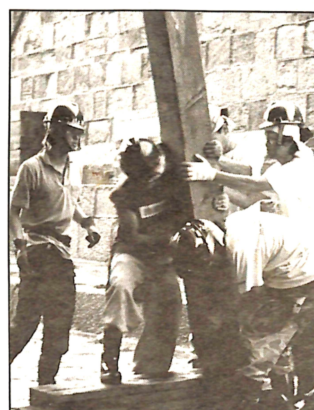
SRF-JRMC employees from shop 68 (Carpenter) installing stern shores.
