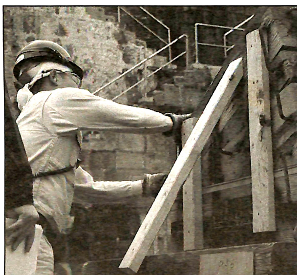
An SRF-JRMC employee checks the positioning of the support blocks before flooding the dry dock.
