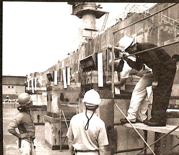
Before allowing water to begin filling the dry dock, SRF-JRMC engineers conduct a detailed verification of support block alignment.
