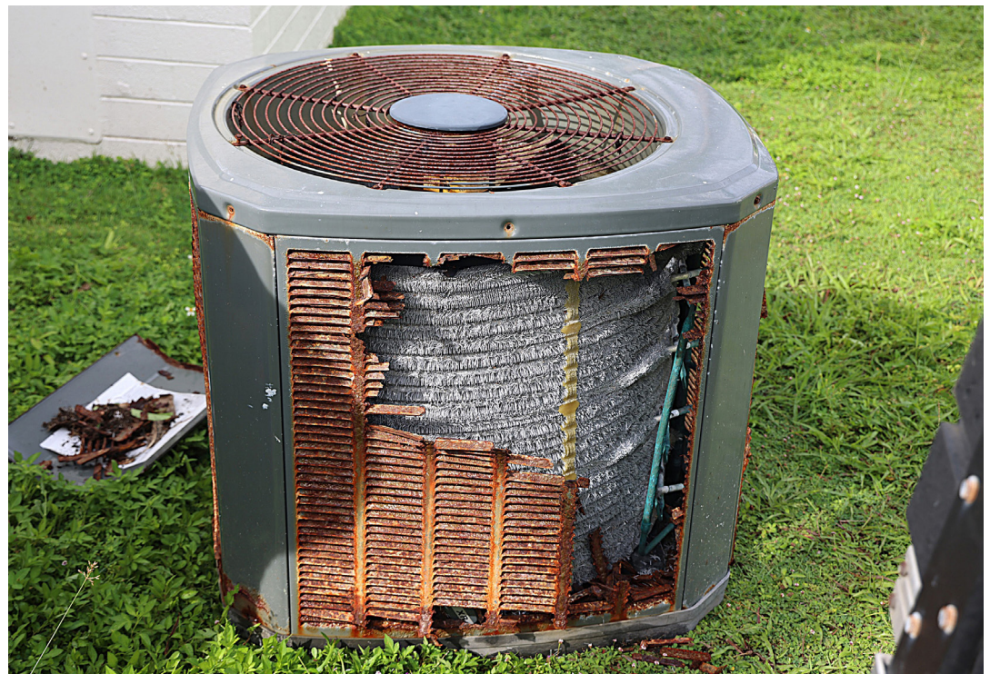
ABOVE: On Kwajalein, AC units (like the one above) often have half the typical U.S. lifespan due to severe climate-driven corrosion.
