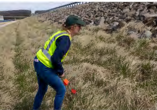
Middle: Geologist Tyler Fox inspects the integrity of the grouted riprap on the upstream right abutment for Hillsdale Reservoirs five-year periodic dam inspection on Tuesday, March 25, 2025.
