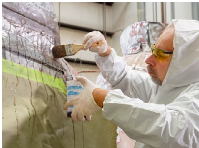
Michael Holguin, Work Leader at the Expeditionary Maintenance Center, applies resin to fiberglass sheets covering newly fabricated metal parts riveted to the body and 10-foot wings of the Fighting Seabee statue.
