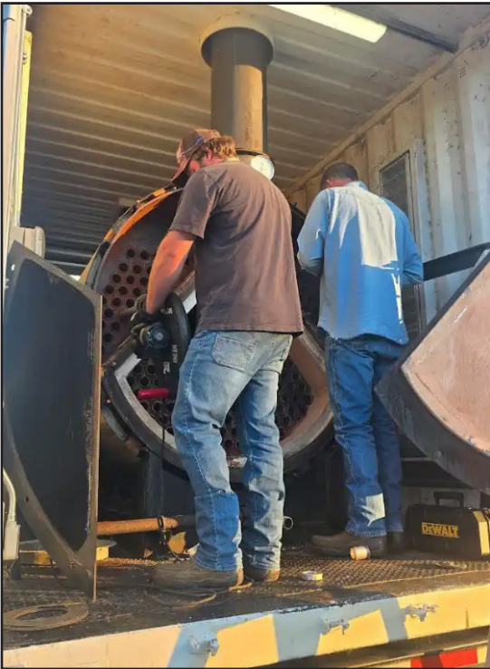
Tyler Cox and Nick Baker with Pine Bluff Arsenal's Directorate of Public Works perform critical maintenance on a high pressure steam boiler. U.S. ARMY PHOTO BY JASON SCHREINER, DPW STEAM AND AIR LEADER
