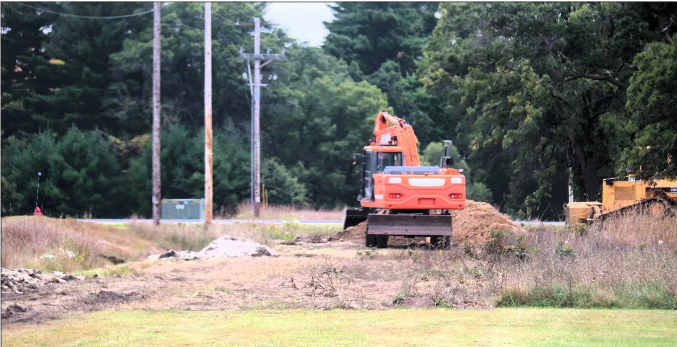
Workers with the installation grounds contractor, Kaiyuh Services LLC, complete work to clear out ditches Sept. 24 at Fort McCoy.
