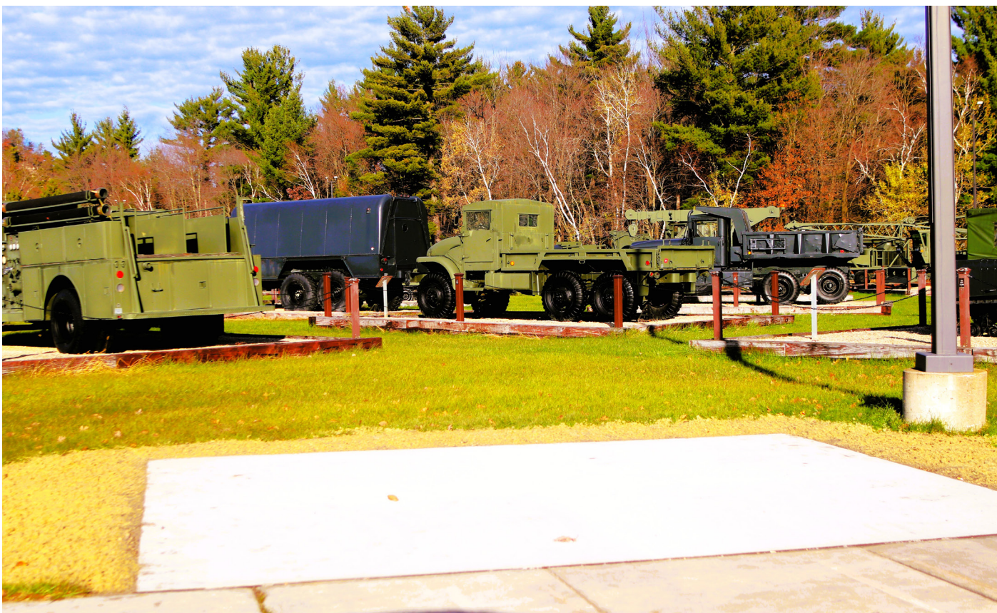
A completed concrete pad is shown at the Fort McCoy Commemorative Area on Nov. 13.
