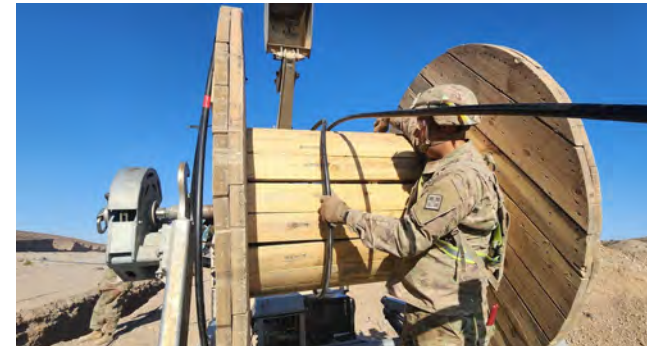
Soldiers from the 712th Engineer Support Company unwind cable to repair a fiber optic cable network at Fort Irwin, Calif. The mission called for trenching and backfilling more than 18,000 feet of rugged desert terrain at multiple sites. (Courtesy photo)
