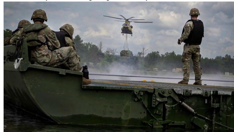
U.S. Army Reserve Soldiers with the 363rd Engineer Battalion conduct bridging operations by connecting bay pieces delivered by a CH-47 Chinook at Global Strike 2025 during the Combat Support Training Exercise (CSTX) at Fort McCoy, Wis., Aug. 7. The CSTX prepares Army Reserve units for deployment by providing realistic, externally evaluated, and collective training scenarios. (U.S. Army Reserve photo by Staff Sgt. Philip Ribas)
