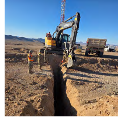
Soldiers from the 712th Engineer Support Company dig trenches for the 812th Tactical Installation and Networking-Enhanced (TIN-E) to inspect and replace fiber optic cable at Fort Irwin, Calif. (Courtesy photo)
