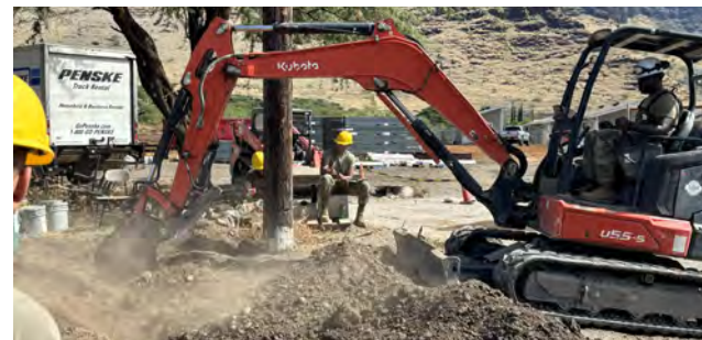
Equipment operators from the 412th Engineer Vertical Construction Company dig utility trenches for plumbing lines. Soldiers were able to maintain their operating skills during their time for this IRT project. (Courtesy Photo)
