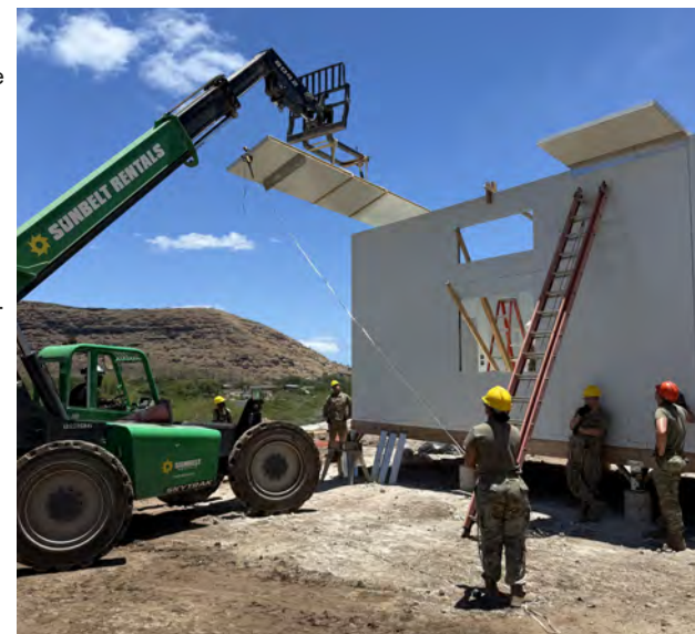
Soldiers from the 412th Engineer Vertical Construction Company guide pieces of a plugin home into place for the Pu'u'honua O' Wai'anae's new site during their annual training July 12-28, 2025. The project is part of the Innovative Readiness Training program that allows units to perform real-world training opportunities through projects that benefit underserved communities. (Courtesy photo)
