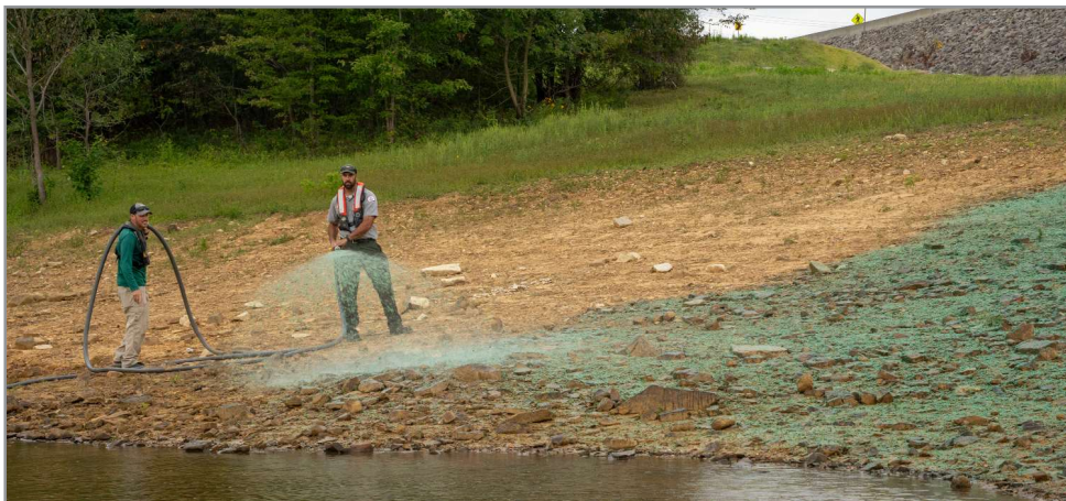
Rough River Lake Park Ranger Adam Taylor and KDFWR's Jeremy Shiflet use a hydro seeder to restore vegetation on eroding shorelines at Rough River Lake in Falls of Rough, Kentucky, Sept. 10.
