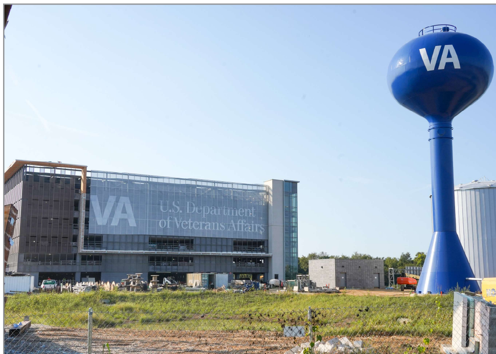
Construction of the new Louisville VA Medical Center in Louisville, Kentucky, is now more than 80 percent complete. Much of that construction included standing up the buildings and facilities across the 34-acre property, but lots of detail work remains to get the project over the finish line.
