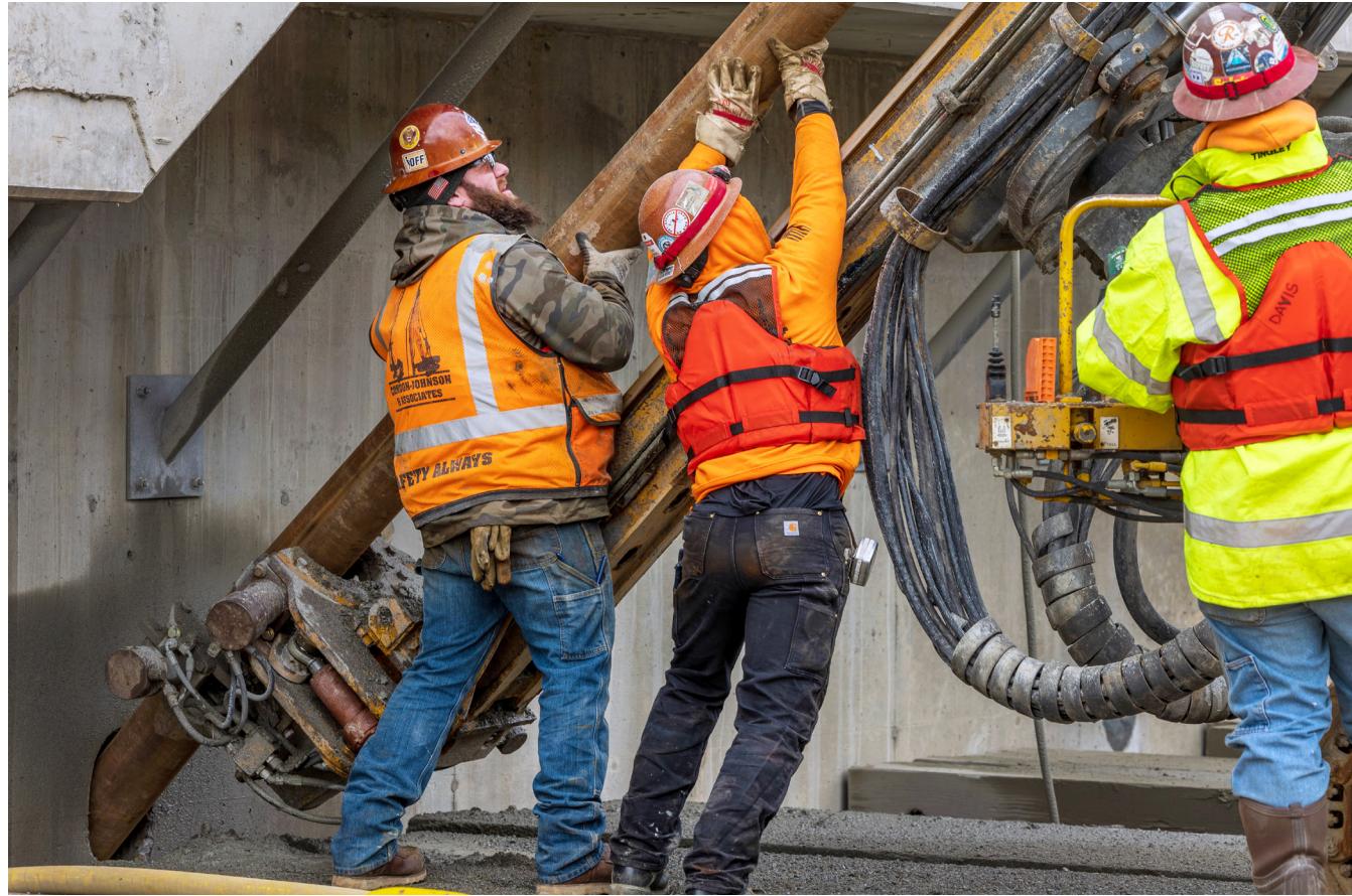
ABOVE: Following an assessment of seismic vulnerabilities, mitigation efforts get underway in Dry Dock 4 at PSNS & IMF, Feb. 9, 2023. Those upgrades will soon continue under a newly awarded $377.7 million contract. (U.S. Navy photo by Wendy Hallmark)
