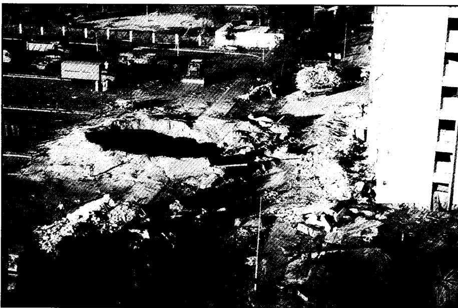
(Top) Outside Khobar Towers, the extent of the destruction is visible. (Bottom) The blast crater as seen from the destroyed civil engineer dormitory building. All photos by Lt. Col. Robbin Schellhous.
