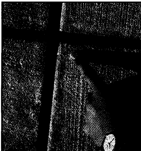
An "excellent" concrete joint. Photos by Tech. Sgt. Eddie C. Riley
