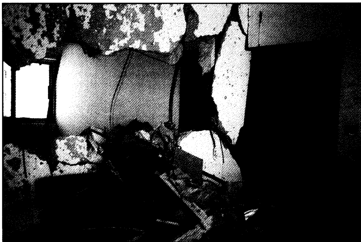
The force of the bomb punched through a six-inch concrete wall and caused the destruction.
