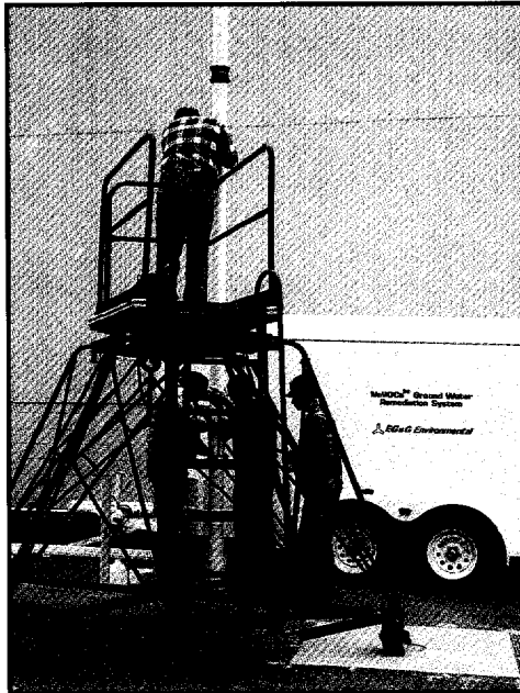
Installing the airlift system
