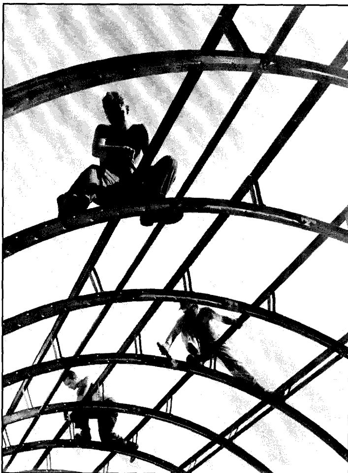
Top - Aviation Engineers place quonset hut ribs on another section of the air base in Marianas. (April 1944)
