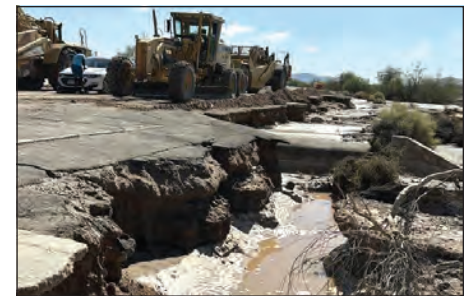
The morning after the Sept. 5 storm, Shearwater's heavy equipment crews were busy doing storm cleanup and repairs. From scrapping to filling in holes, the crews were immediately on the scene getting the area along Imperial Dam Road between the Howard and the Walker gates back in drivable condition. (Loaned photos)
