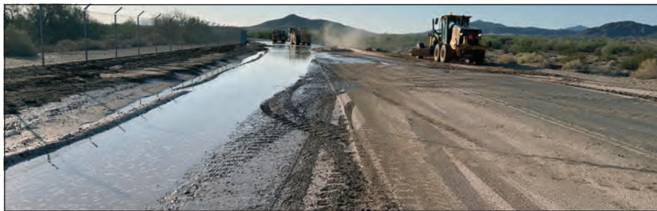
The morning after the Sept. 5 storm, Shearwater's heavy equipment crews were busy doing storm cleanup and repairs. From scrapping to filling in holes, the crews were immediately on the scene getting the area along Imperial Dam Road between the Howard and the Walker gates back in drivable condition. (Loaned photos)
