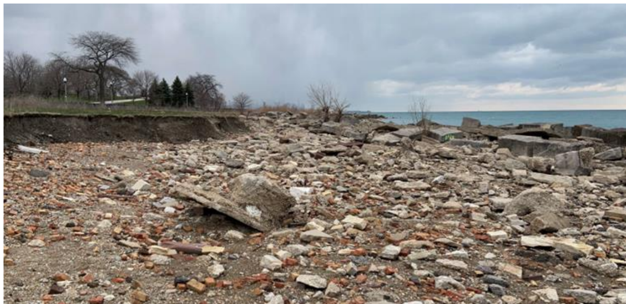
Figure 3: Erosion of parkland behind failed timber cribs and displaced limestone blocks
