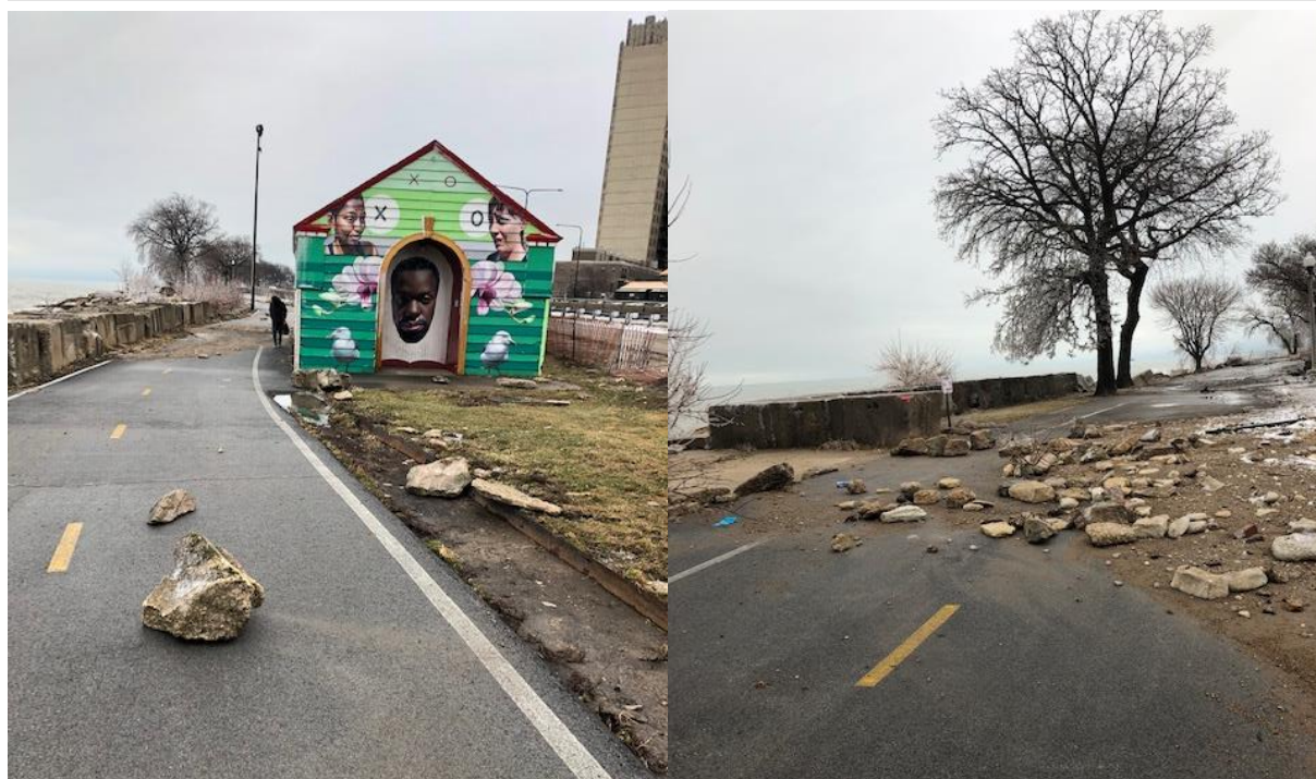
Figure 44: Rock ejecta on the Lakefront trail after the January 11, 2020 storm as an example of continued coastal threats with the no action alternative.
