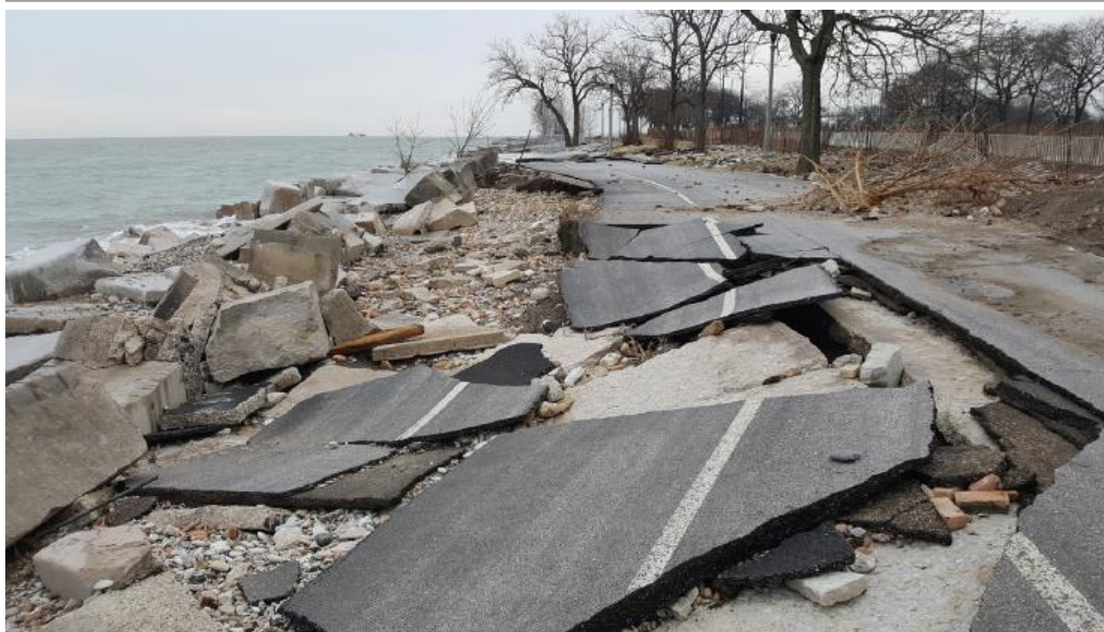
Figure 43: Damage to the revetment and Lakefront Trail in the Morgan Shoal reach of the Chicago shoreline from a storm on January 11, 2020.
