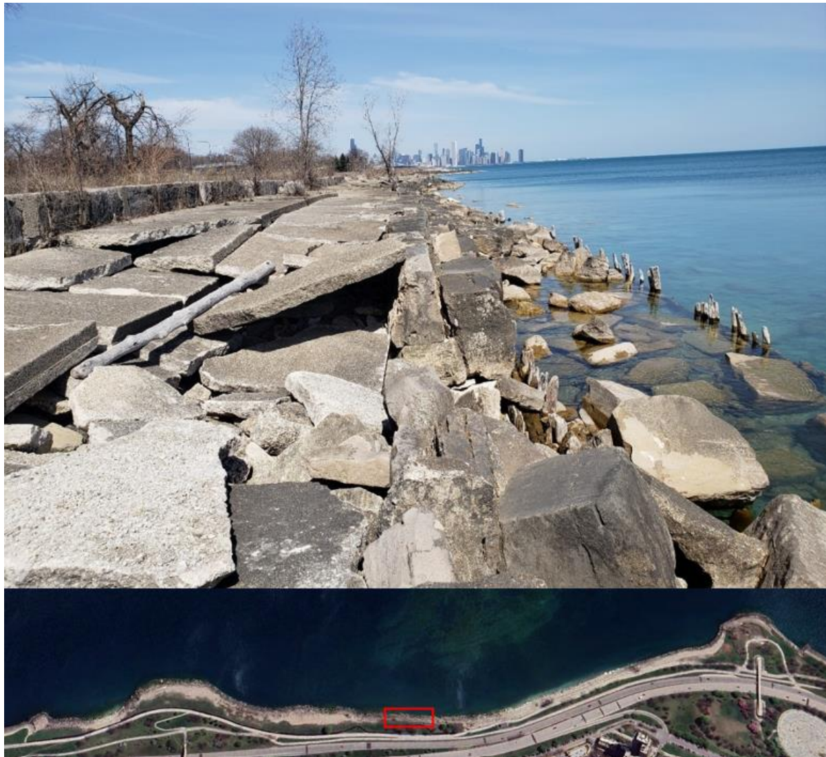
Figure 11: Deteriorating pedestrian promenade and revetment with exposed deteriorated timber cribs along the Morgan Shoal reach which has experienced structural failure, looking north (March 2023). Reference box (red) indicating location of photo (bottom).
