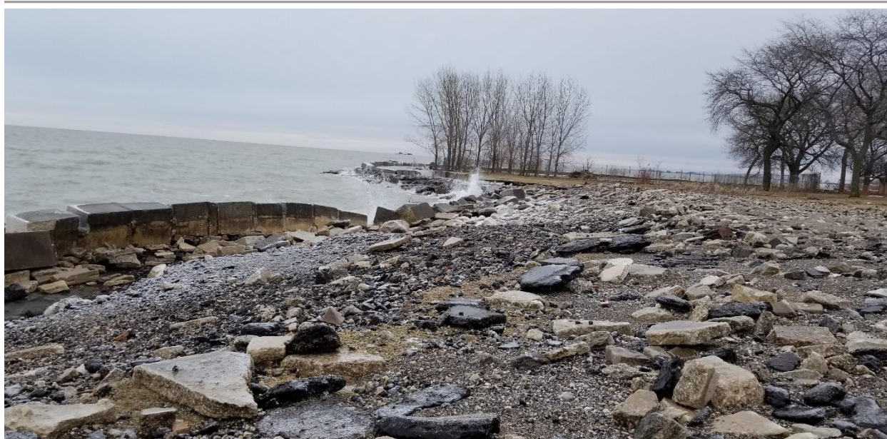
Figure 28: Backshore erosion and land loss with failing revetment. Photo after January 2020 storm as an example of continued erosion under the no action alternative.
