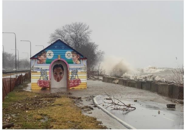
Figure 2-6. Inundation of the washroom building and pedestrian Lakefront Trail at 49 th Street during the January 11, 2020 storm event.
