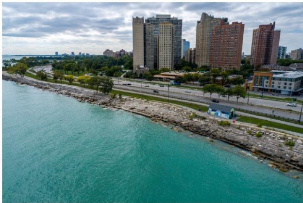
Figure 2-3. View of central portion of project site, looking south. The existing washroom building and the paved beach are visible, as is the nearby DuSable Lake Shore Drive. This area is the narrowest portion of Burnham Park and has been repeatedly damaged by storms.
