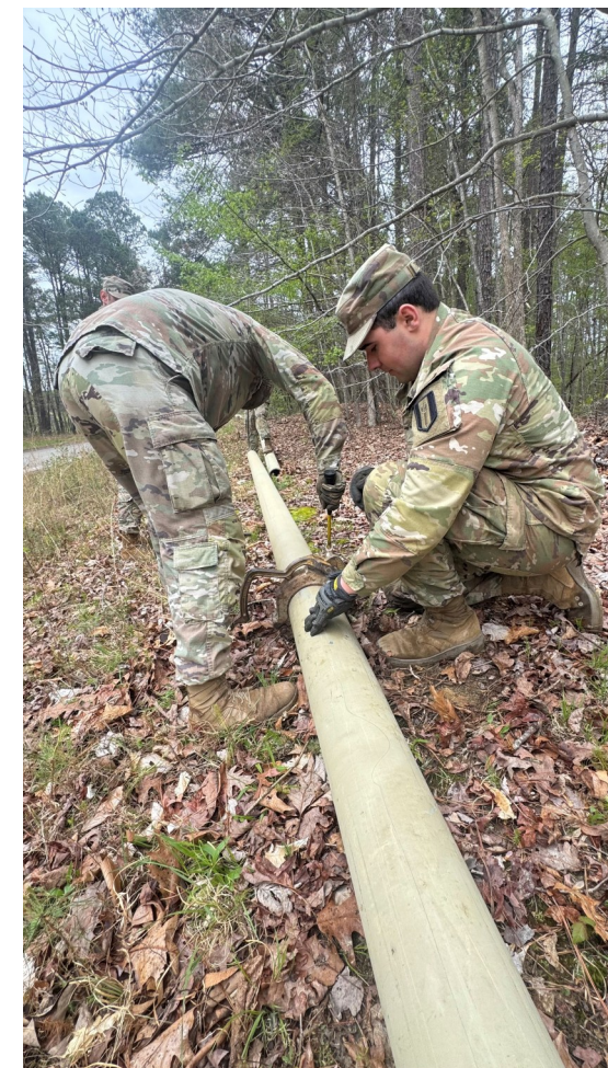
Engineers from the 368th Engineer Battalion line up two sections of pipe and connect them with a coupler. (Courtesy Photo)
