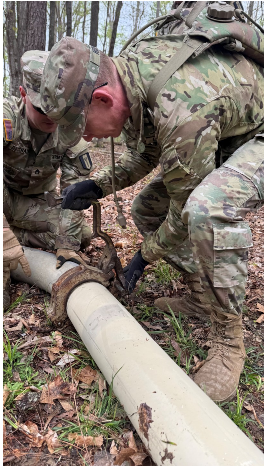
Engineers begin to lock in two sections of pipeline with a coupler. (Courtesy Photo)
