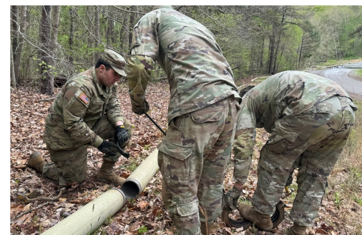
Soldiers gathering coupling before connecting two sections of pipe. (Courtesy Photo)
