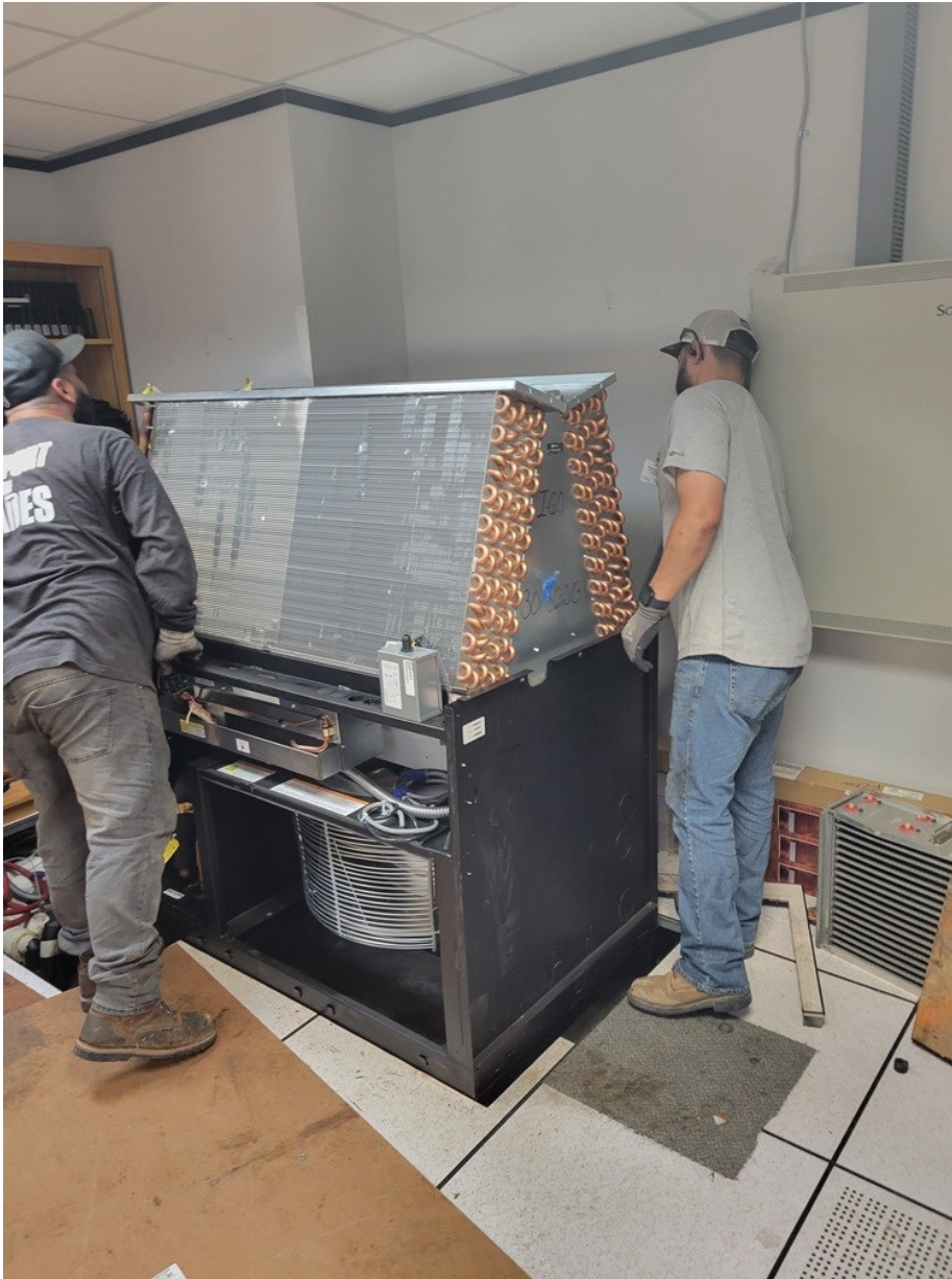
Contractors set the coils into the Liebert AC unit during assembly. (Courtesy photo.)
