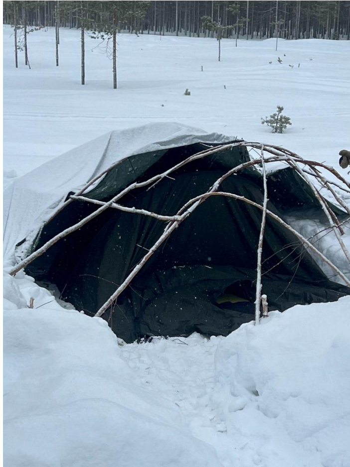
Birch lattice over Squad tent for heat standoff.
