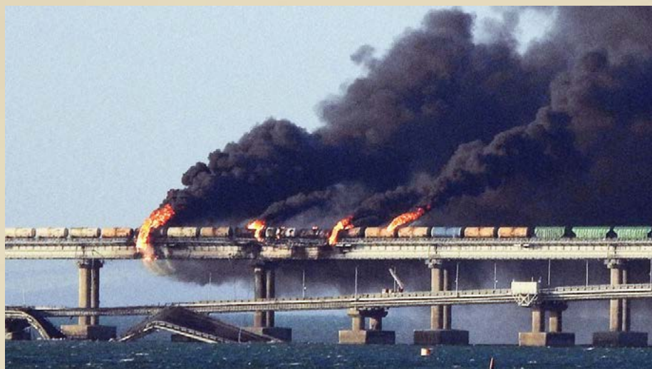
October 2022 attack on Kerch Straits Bridge
