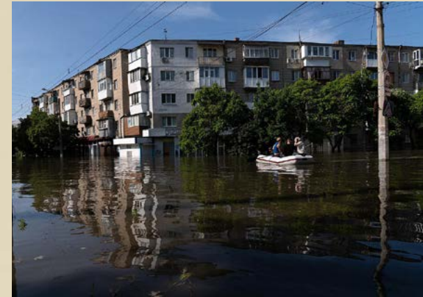
Kherson the day after the destruction of the Kakhovka Dam (State Emergency Services Ukraine)
