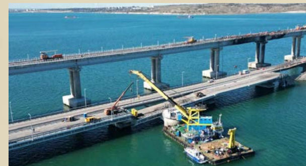
Repairs on Kerch Strait Bridges
