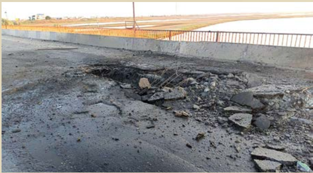
Chonhar Bridge in occupied Crimea (Telegram)
