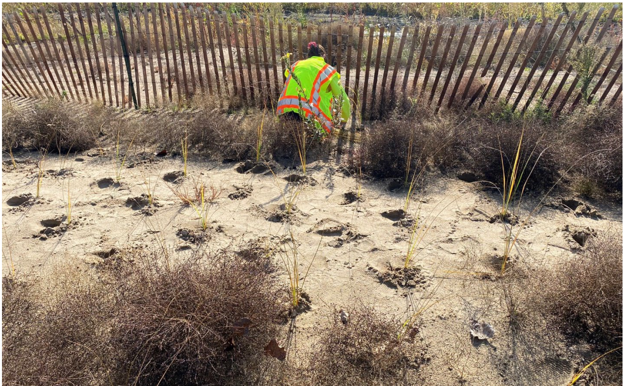
Photograph 12: Post-construction planting of native dune vegetation (looking south towards East Perry Street) (2022)
