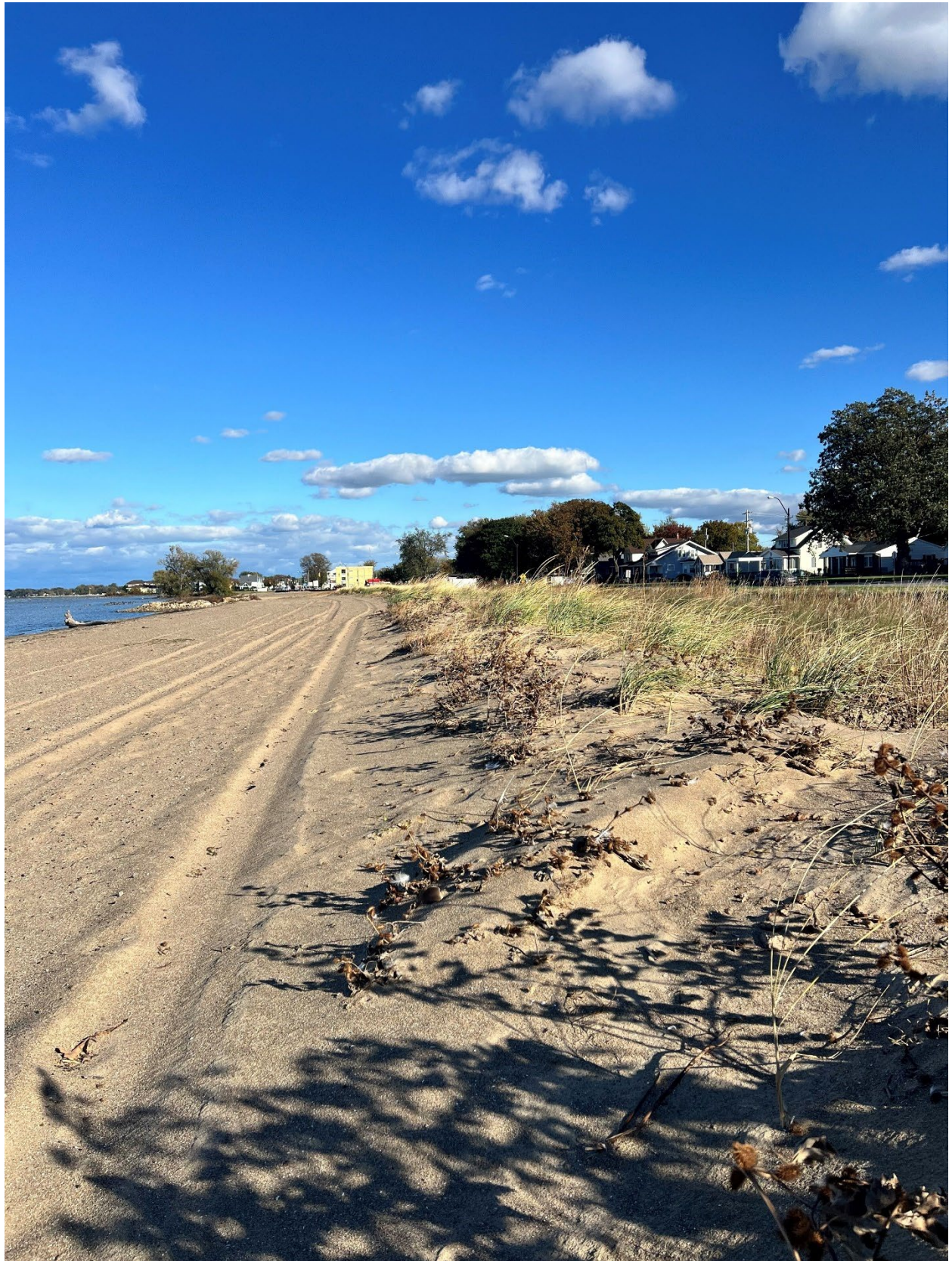
Photograph 18: Post-construction planted dunes (Looking east from Lake Erie Shoreline) (2024).
