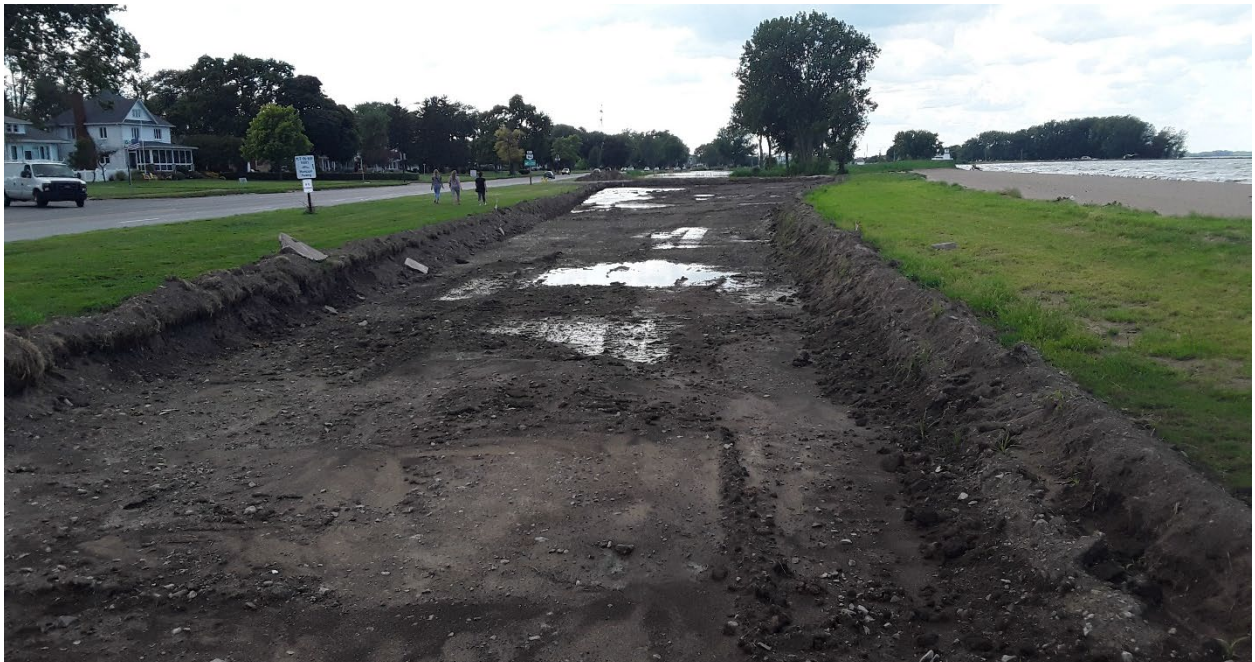
Photograph 8: Construction photo within the wetland extension (looking west towards the existing wetland and Waterworks Park) (2020).
