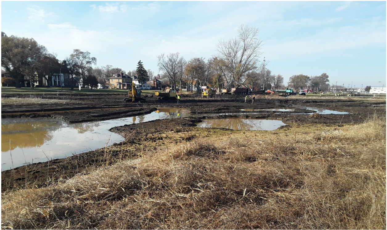
Photograph 5: Construction photo within the existing wetland (looking west towards East Perry Street and Waterworks Park) (2019).
