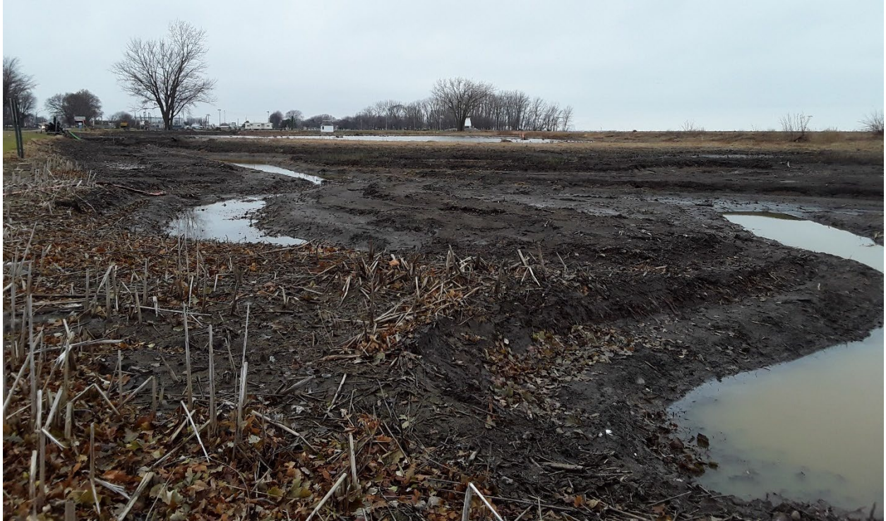
Photograph 7: Construction photo within the existing wetland (looking west towards Waterworks Park) (2019).
