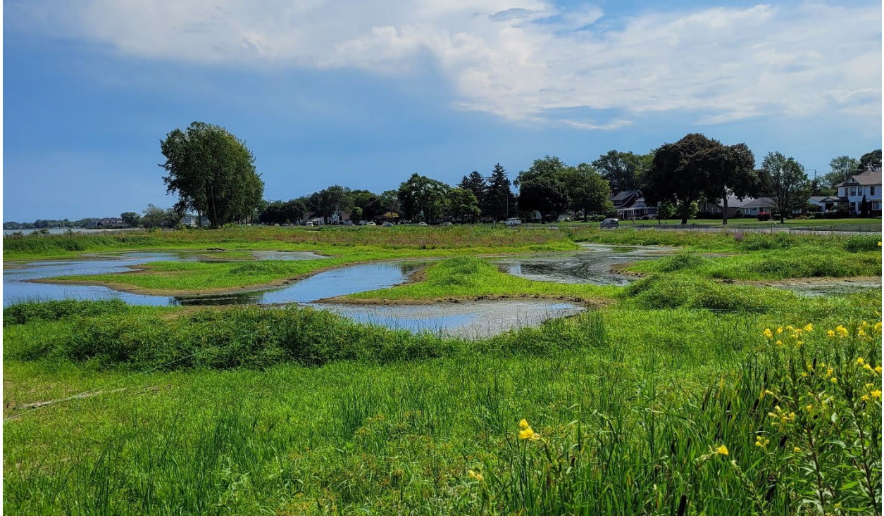
Photograph 13: Post-construction (looking east from Waterworks Park) (2023).
