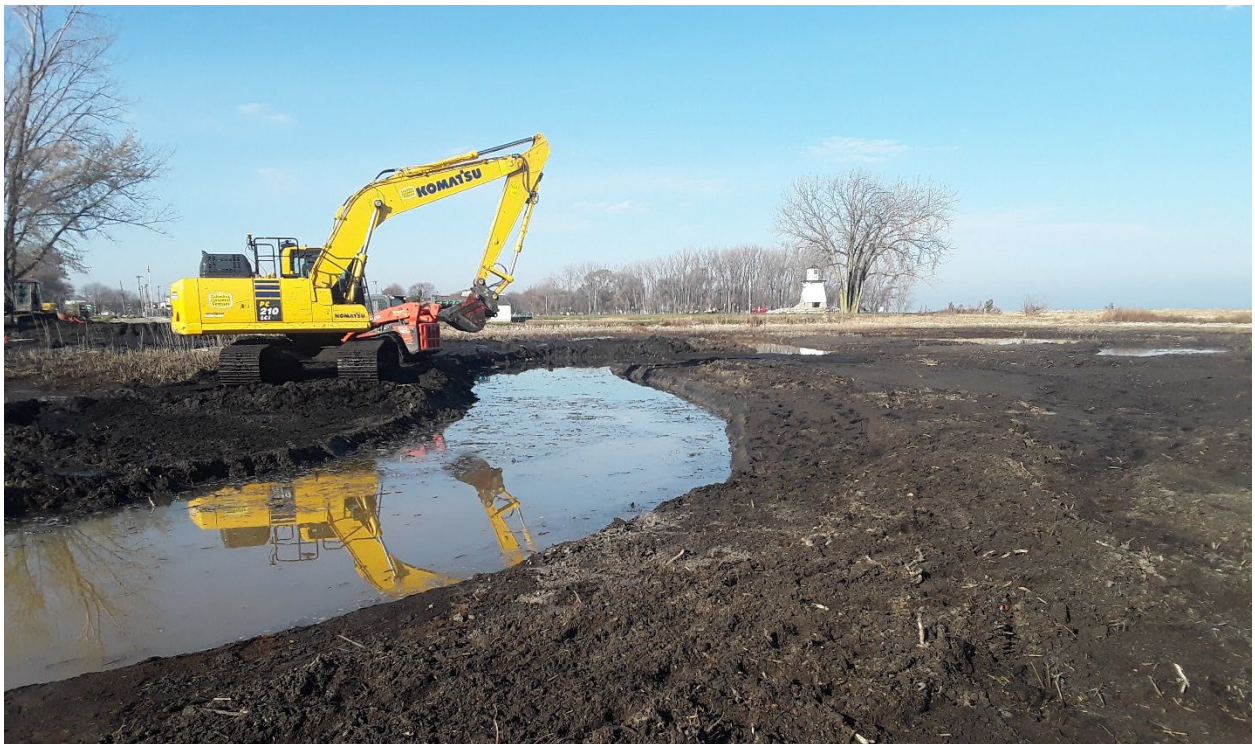
Photograph 6: Construction photo within the existing wetland (looking west towards Waterworks Park) (2019).
