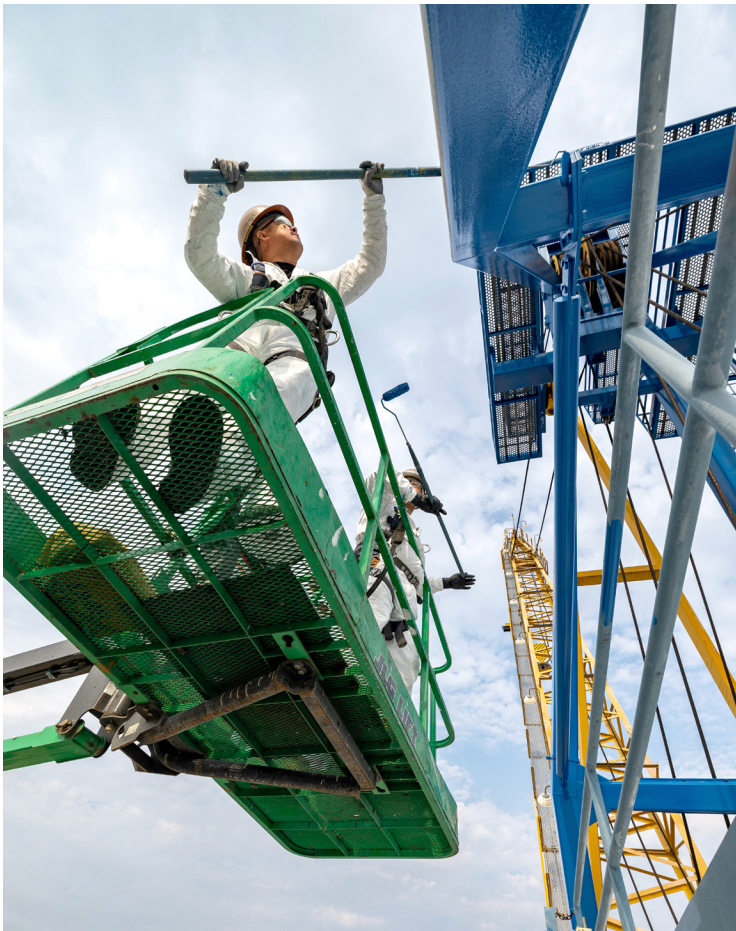
ABOVE: Darius Aldan, work lead, and Romeo Aquino, painter, Code 730, Crane Maintenance, are part of six-person team repainting Portal Cranes 80, 82 and 92. (U.S. Navy photo by Wendy Hallmark)
