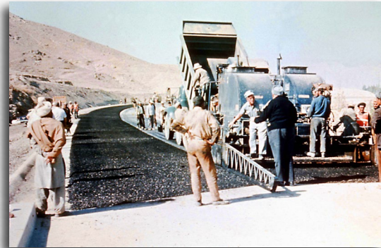
Afghan highway asphalt laying Early 1960s
