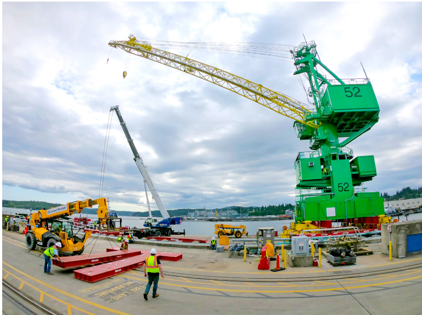
ABOVE: Code 700, Lifting and Handling, team members begin moving the 255-foot tall Crane 52 from its barge to the tracks at PSNS & IMF, July 14. The crane is the first of two new cranes set to aid shipyard operations. (U.S. Navy photo by Jeb Fach)
