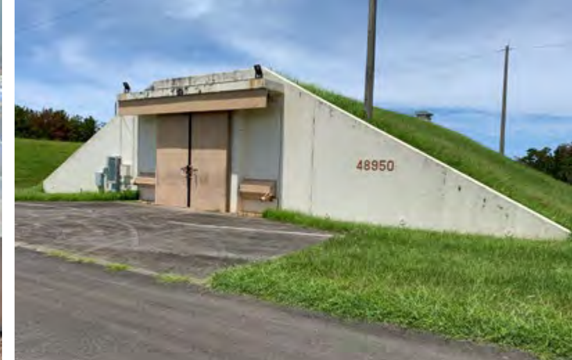
Earth-Covered Magazine at Kadena Air Base, Japan.
