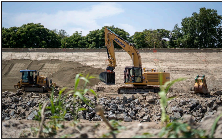
An excavator smooths bedding material May 1 on the slope of a levee in Riverside, California, where the U.S. Corps of Engineers Los Angeles District, Riverside County Flood Control and Water Conservation District and contractors have started work again for the levee rehabilitation project.
