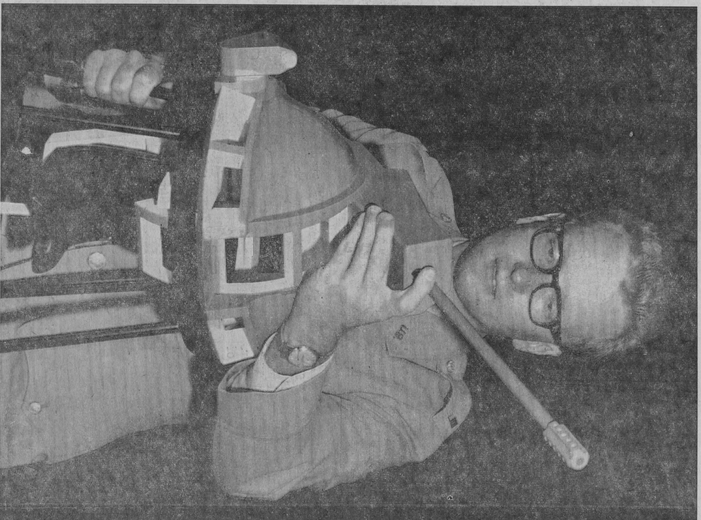
CUPOLA CONCEPT — Lt. Allan Galbavy holds gun mount of one-quarter scale model of one-man cupola, related in design to family of animal having jointed appendages and horny external skeleton. Galbavy, who was assigned to future weapons design, worked on bionics studies before leaving the Army recent ly.
