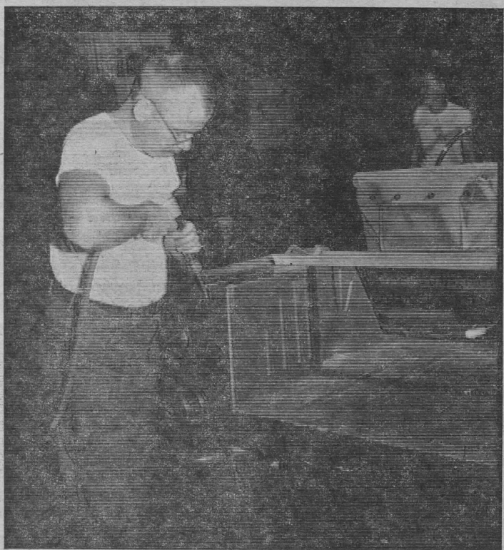
EARLY STEP — Harry Moorman demonstrates first major step in modifying jeeps — cutting away metal of standard model to make room for weapon mounting brackets. He's using pneumatic edging cutter that slices metal easily.
