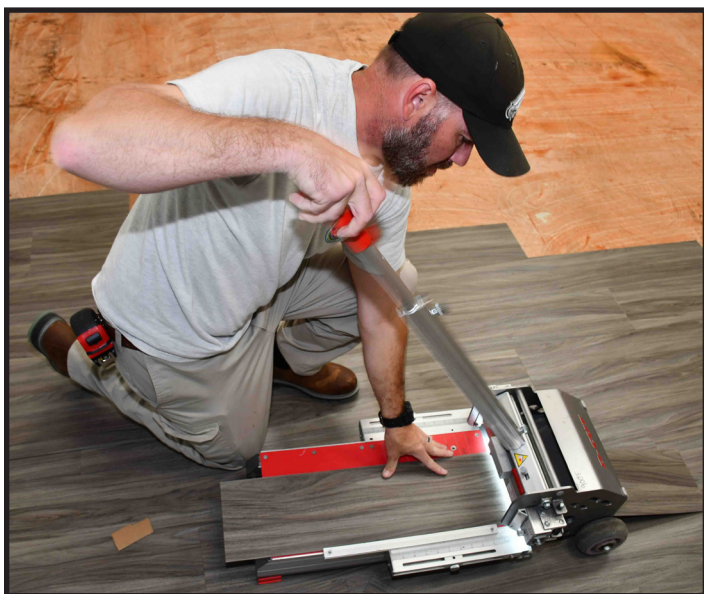
From left to right: Code 900F.41 Maintenance Mechanic Brian Sumner trims floor tiling for a recent renovation for the Information Technology and Cybersecurity Department (Code 109) IT Customer Service Desk and office space areas; Code 900F.41 Maintenance Mechanic Cody Tucker lays down tile for a recent renovation for the Code 109 IT Customer Service Desk and office space areas.
