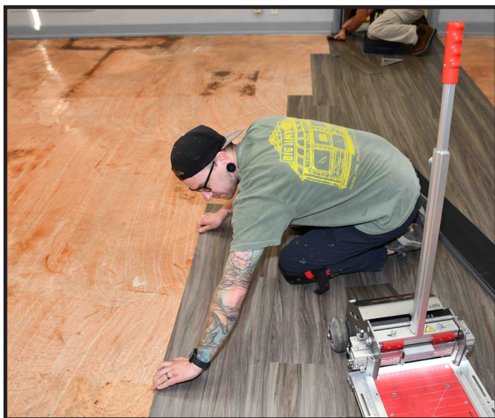
From left to right: Code 900F.41 Maintenance Mechanic Brian Sumner trims floor tiling for a recent renovation for the Information Technology and Cybersecurity Department (Code 109) IT Customer Service Desk and office space areas; Code 900F.41 Maintenance Mechanic Cody Tucker lays down tile for a recent renovation for the Code 109 IT Customer Service Desk and office space areas.
