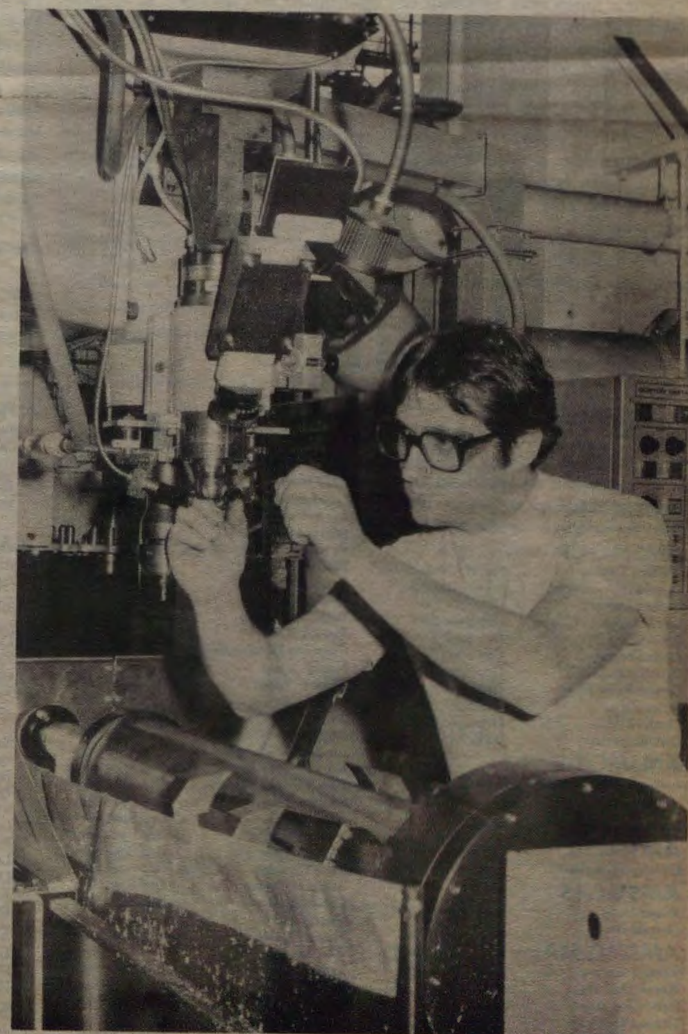
Machinist Wayne Richardson adjusts the light source on an RIA milling machine equipped with a computerized sensing device and control system. In addition to milling metal, the machine also performs a complete quality assurance inspection. The machine is about five years ahead of other state-of-the-art machine tools.
