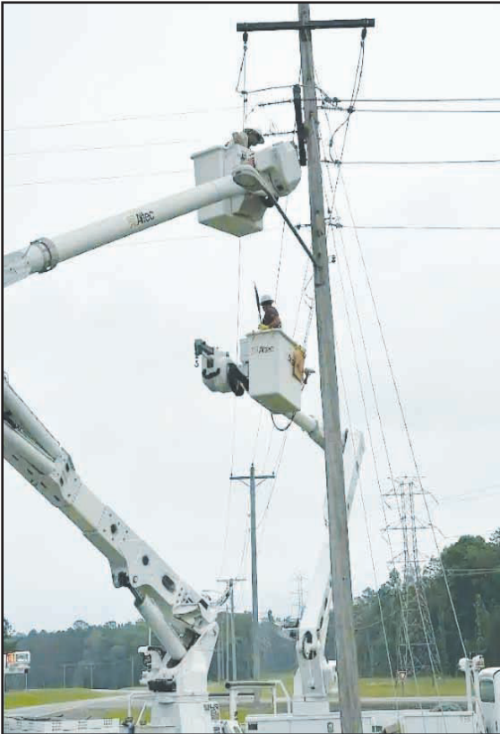
Wes Hoffman and Ryan Garrett with Pine Bluff Arsenal's Directorate of Public Works-Electric Shop repair high-voltage power lines following recent storms. U.S. ARMY PHOTO BY CAITLIN THOMAS-DPW
