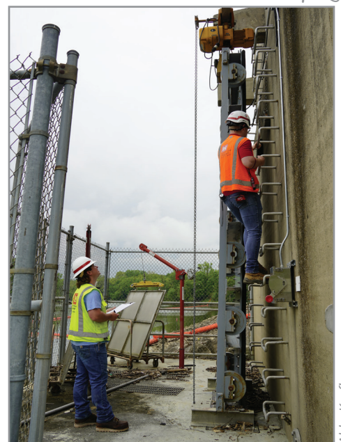
Louisville District structural engineers conduct a Hydraulic Steel Structure (HSS) inspection of the emergency gate at West Fork Lake, May 14, 2025.
