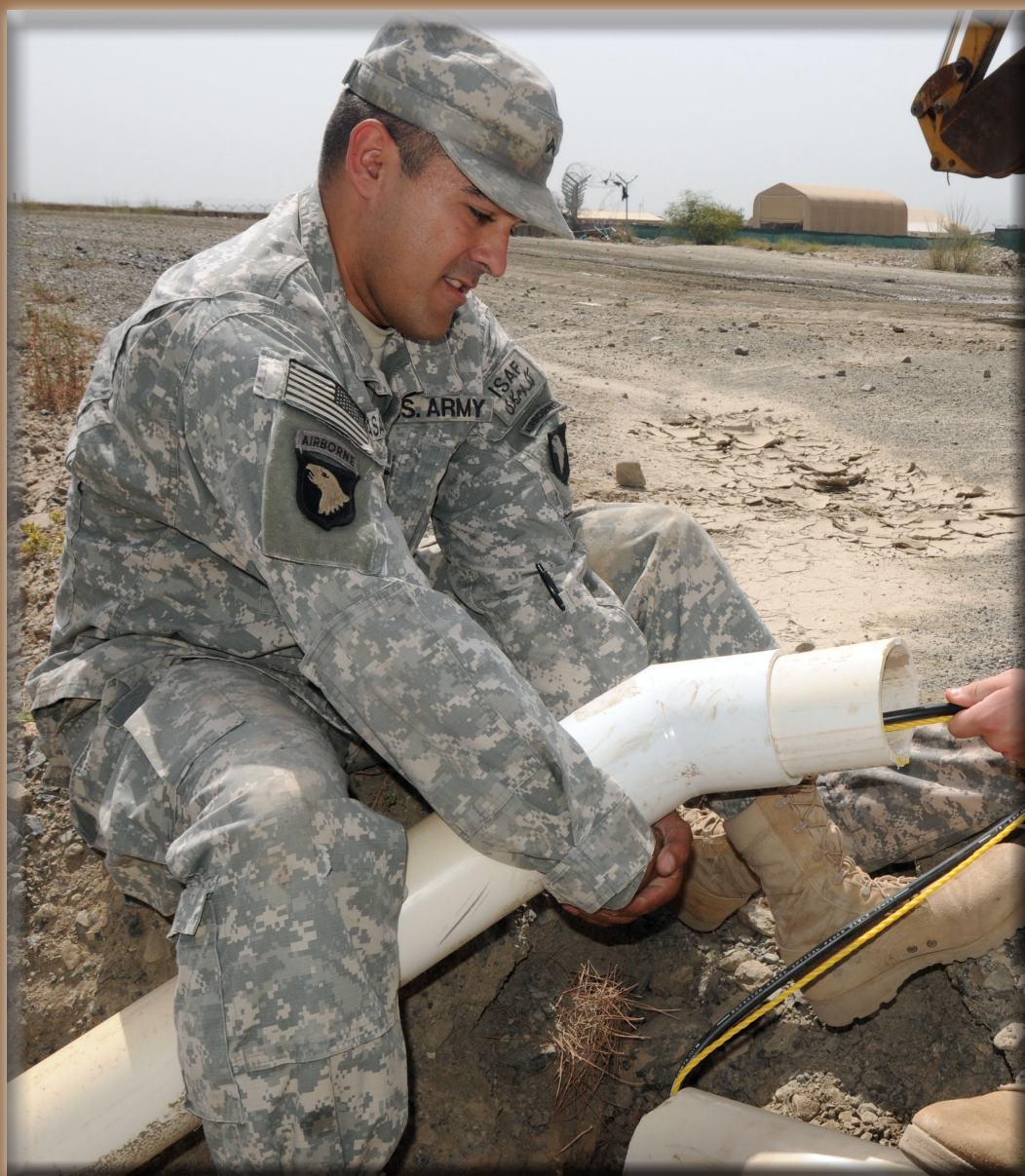
(Above) Cpl. Luis A. Casanadelapaz, C Co, 3 rd STB holds plastic piping steady while another person pulls a black and yellow fiber optic cable through it. (Right) Spc. Maria Hazel Pagan, C Co., 3 rd STB uses a pair of pliers to hold fiber optic cable.
