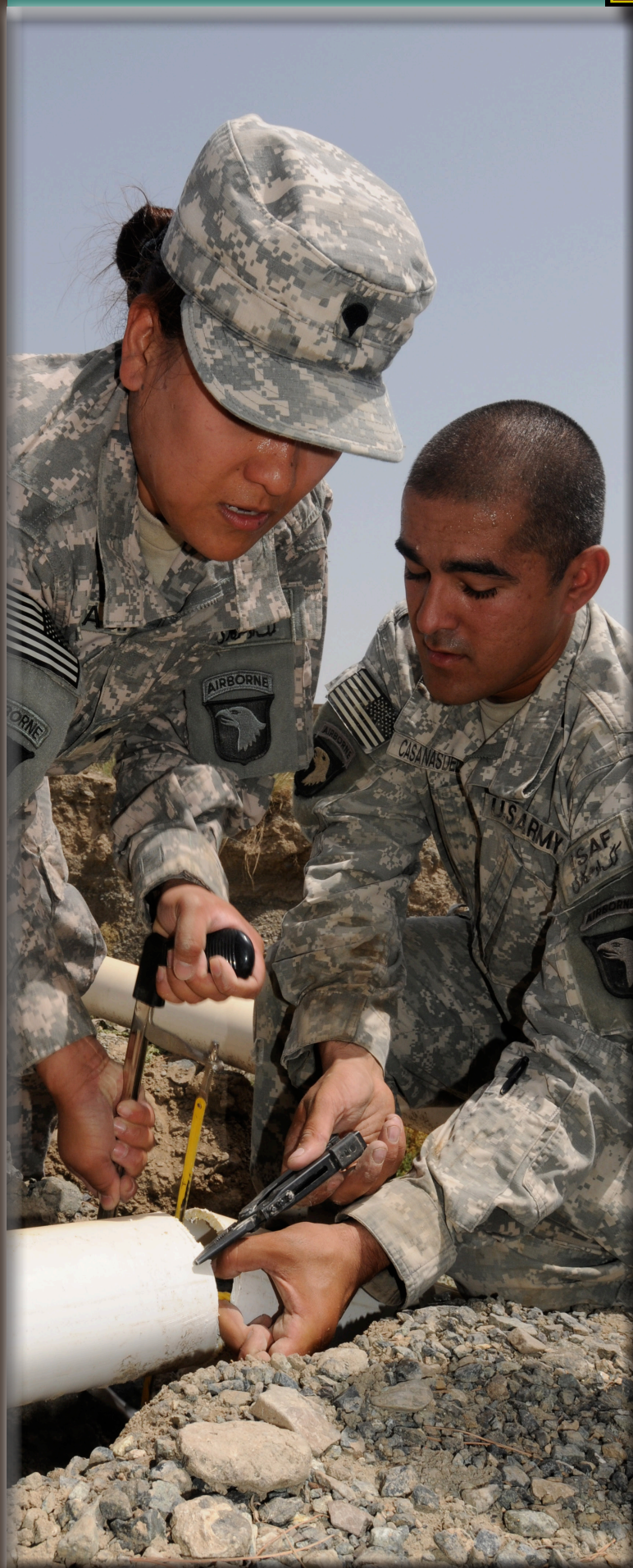
While Spc. Andrew T. Lanham, C Co., 3rd STB, pulls fiber, another soldier uses a hacksaw to saw through a plastic pipe while Cpl. [name obscured] cable and rope out of the way.
