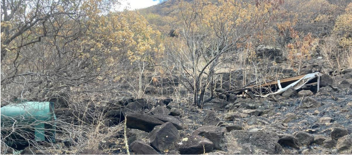
Catchment with gutter and hoses melted by the fire
