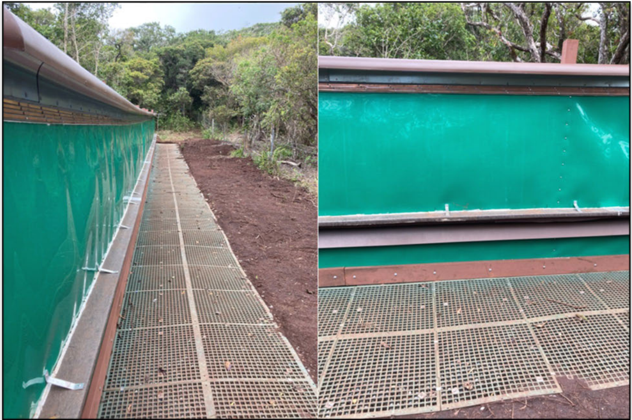
Figure 3: Kahanahaiki enclosure design: two views of the outside wall with predator barriers. Barriers include the rat hood at the top and electric wires, cut mesh and angle for E. rosea .
