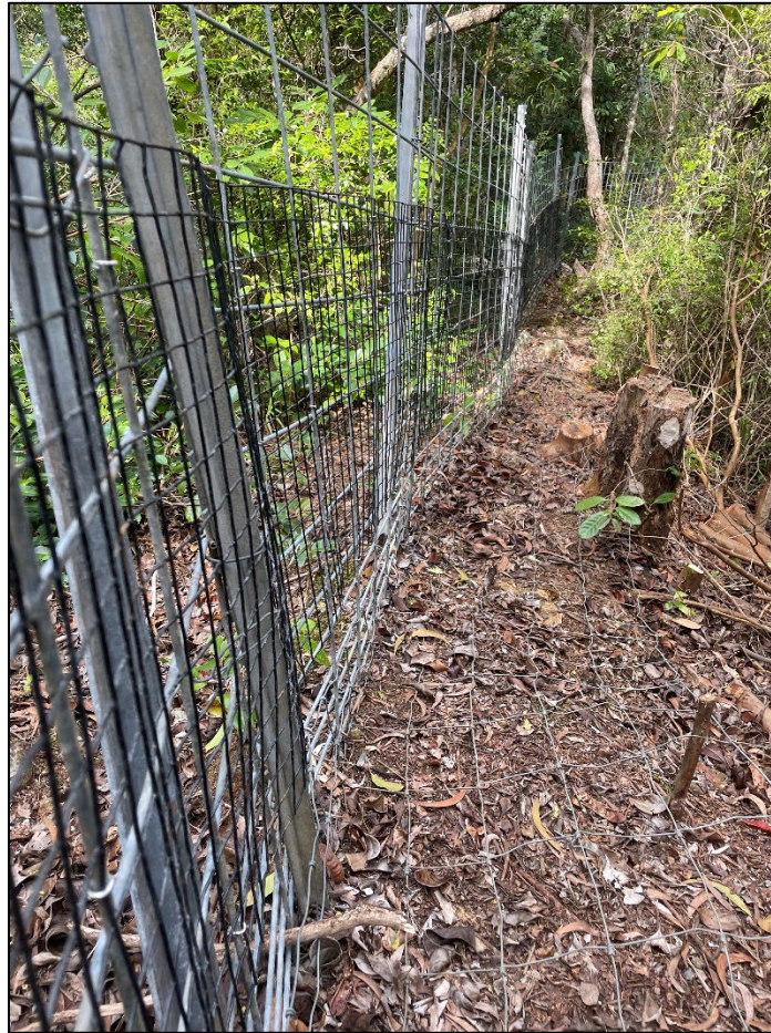
Figure 3: Fickle wire (black mesh) attached to the bottom of cattle panel fence.
