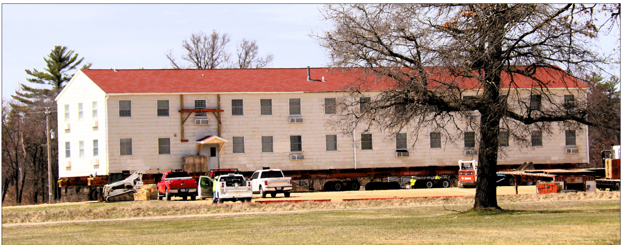
(Above and below) A barracks building from the 1600 block at Fort McCoy is shown being moved April 16 from the 1600 block to another area of the installation. This was fourth building move since work started in January. Devooght Building Movers of Manitowoc, Wis., is the contractor doing the building moving.
