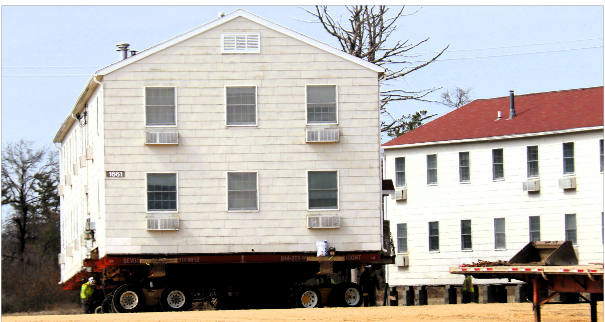
(Above and below) A barracks building from the 1600 block at Fort McCoy is shown being moved April 16 from the 1600 block to another area of the installation. This was fourth building move since work started in January. Devooght Building Movers of Manitowoc, Wis., is the contractor doing the building moving.
