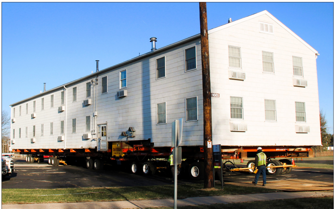
(Above and below) A barracks building from the 1600 block at Fort McCoy is shown being moved April 16 from the 1600 block to another area of the installation. Contractors are moving several buildings in 2025. These buildings will eventually be reset at another area of the post so new construction can begin in their current location on new officer quarters.
