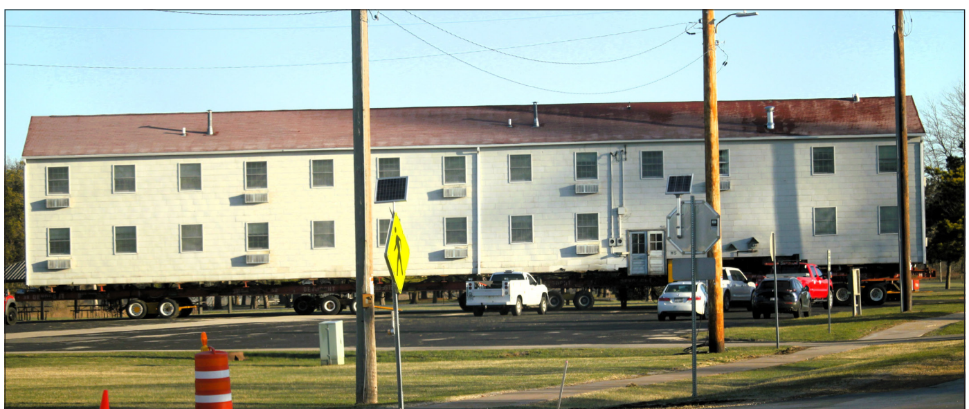
(Above and below) A barracks building from the 1600 block at Fort McCoy is shown being moved April 16 from the 1600 block to another area of the installation. Contractors are moving several buildings in 2025. These buildings will eventually be reset at another area of the post so new construction can begin in their current location on new officer quarters.
