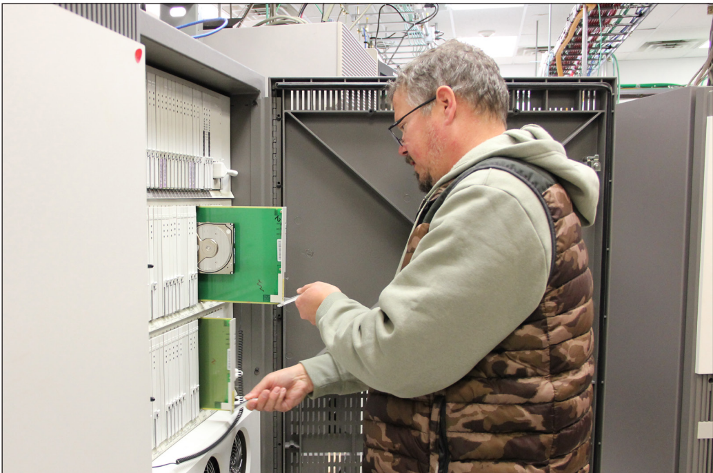
Fort McCoy Network Enterprise Center employee Kenneth O'Connell disconnects the last legacy Time Division Multiplexing equipment for telecommunications Nov. 21, 2024, at Fort McCoy. Fort McCoy changed its telecommunications to voice over internet protocol in 2024.
