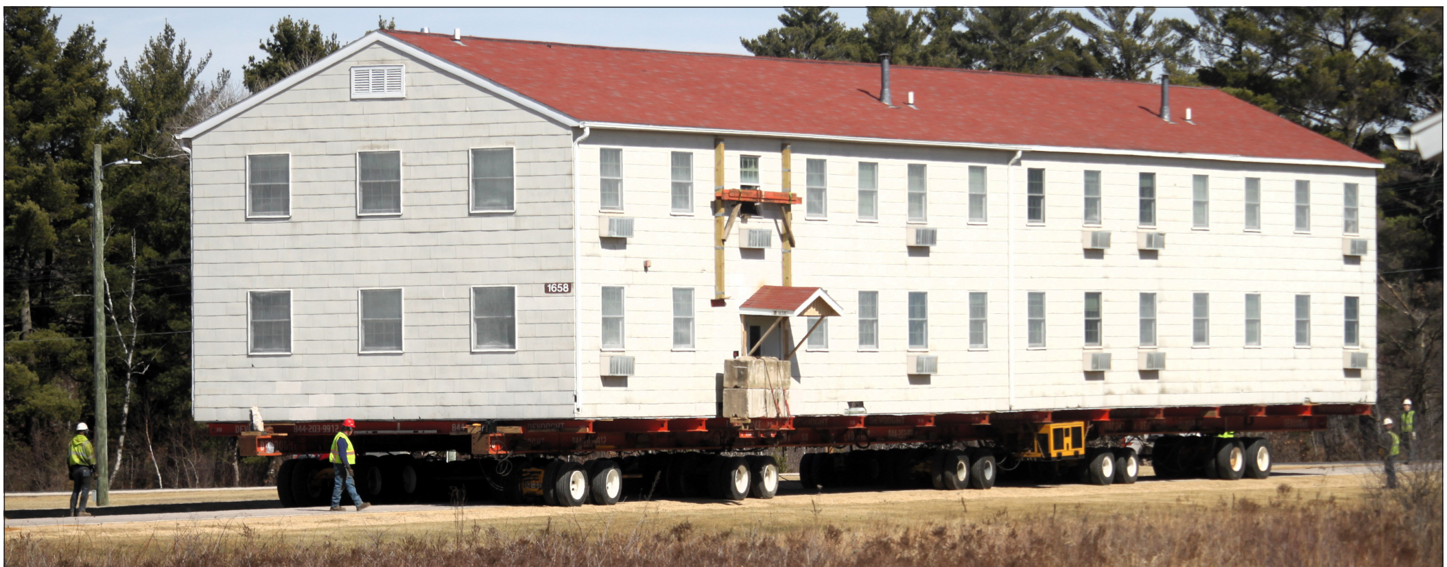
A barracks building from the 1600 block at Fort McCoy is shown about half-way through its move March 18 from the 1600 block to the 500 block of the installation.
