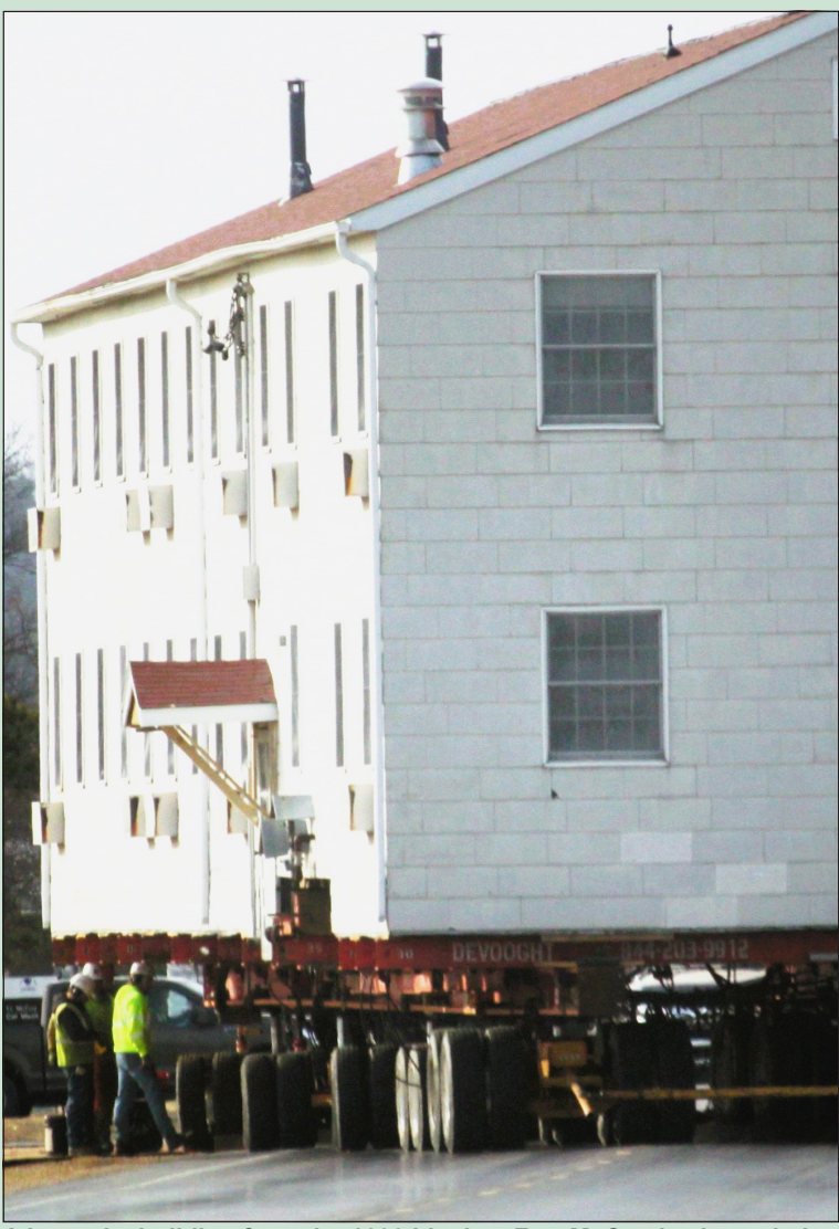
A barracks building from the 1600 block at Fort McCoy is shown being moved March 18 from the 1600 block to another area of the installation.
