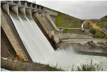
Water releases at Folsom Dam, Calif. (Credit: U.S. Bureau of Reclamation)
