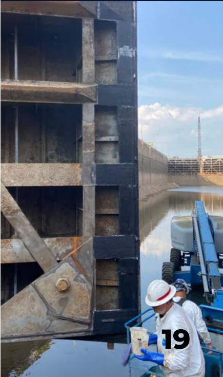
CW RD&T partners with USACE Districts to transition Fiber Reinforced Polymer innovations for Hydraulic Steel Structure projects.
