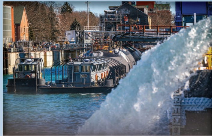
Dry Dock 1 and the Superflood Basin are being flooded in preparation for USS Cheyenne (SSN 773) undocking.
