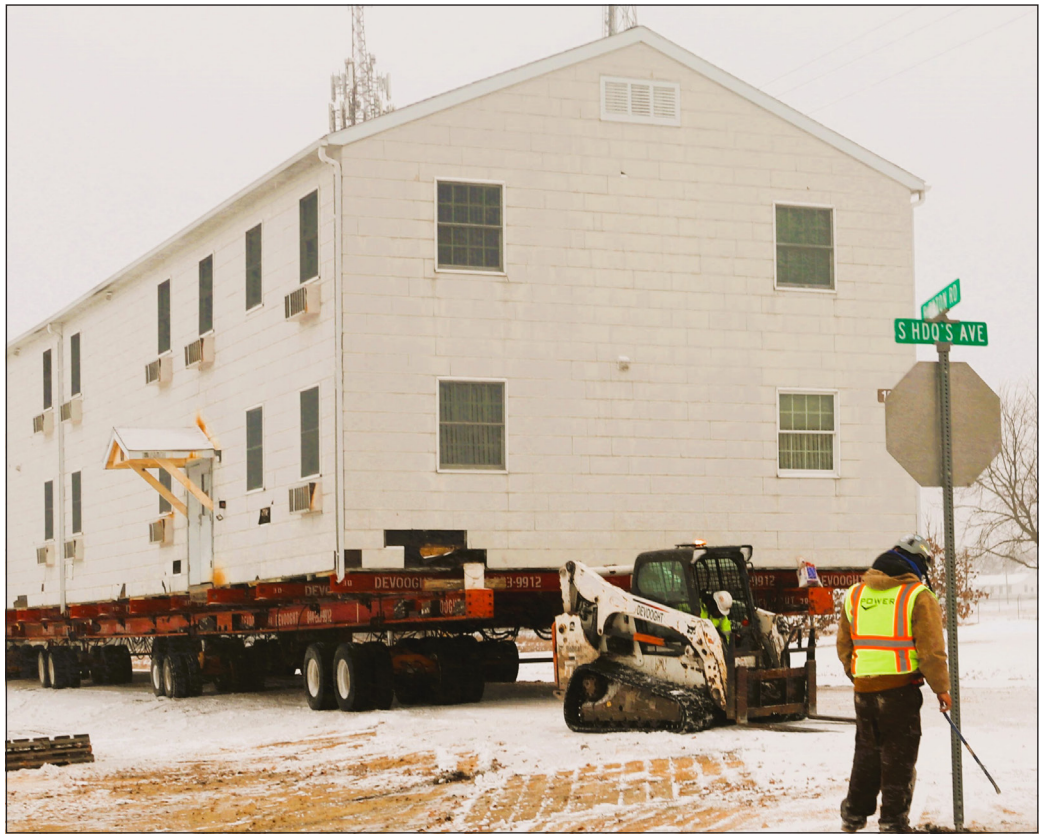
(Above and below, all photos) Contractors move the second of five World War II-era barracks from the 1600 block at Fort McCoy on Feb. 13 to another area of the installation.
