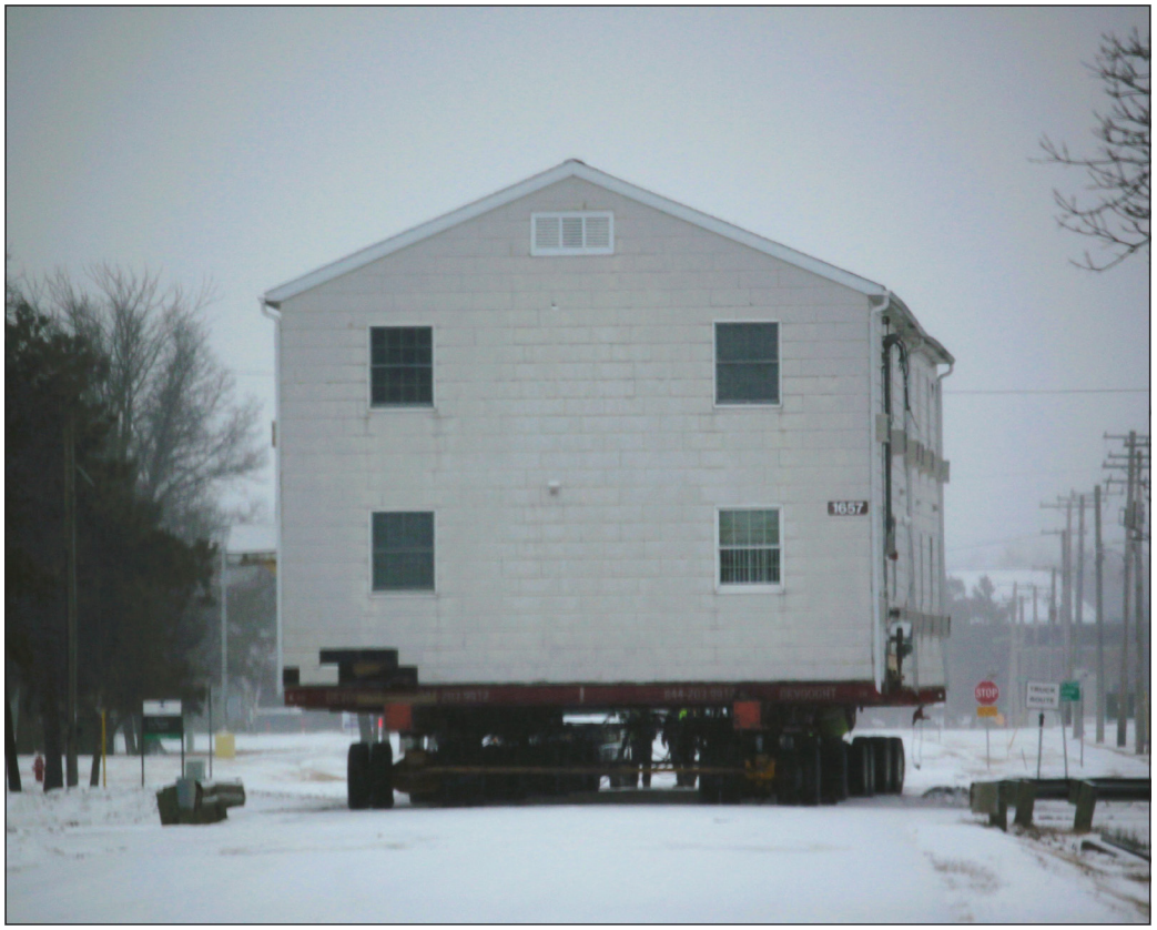
(Above and below, all photos) Contractors move the second of five World War II-era barracks from the 1600 block at Fort McCoy on Feb. 13 to another area of the installation.
