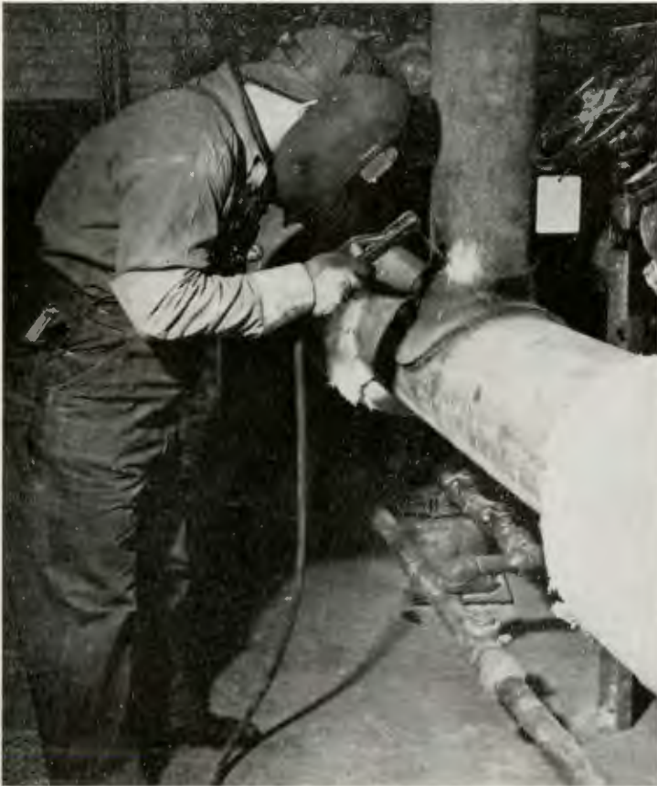
Roy Hartman, Maintenance Department, does pipe welding job.
