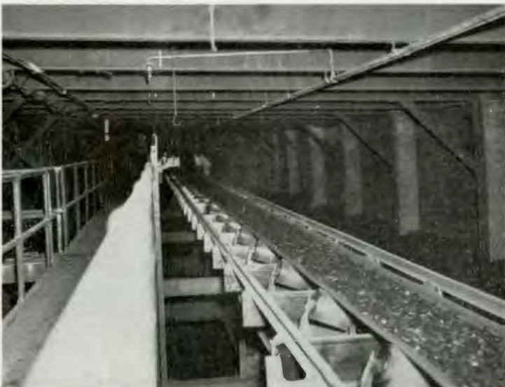
Coal conveyor in boiler house. This Gargantua moves 60 ton per hour.
