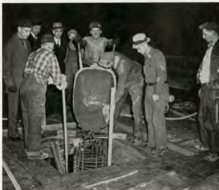
Pouring a concrete column for a new addition to old Forge Shop.
