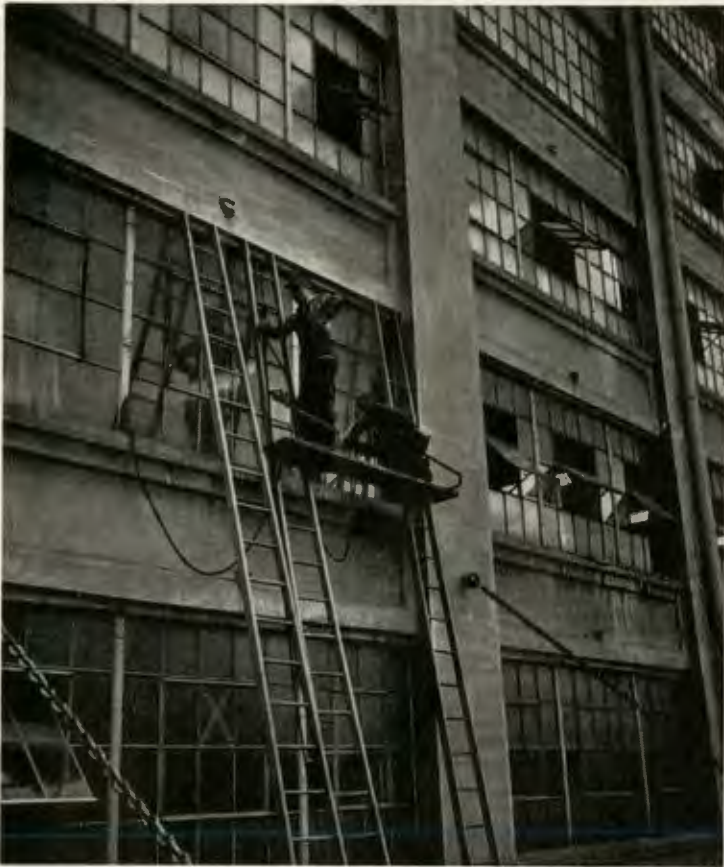
Neal Harrah (standing) and J. P. Dokas (welder) repair a steel sash.
