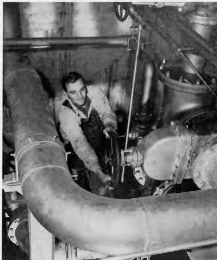
Walter S. Bell regulates the amount of compressed air to leave the air compressor plant through this piping. The compressed air is used to drive tools, hoists, sand blast and other pneumatic equipment.
