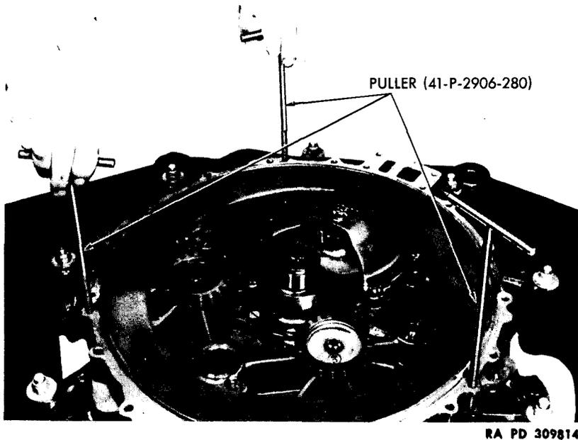
*Figure 51 – Removing Crankcase Diffuser Section From Rear Section*
